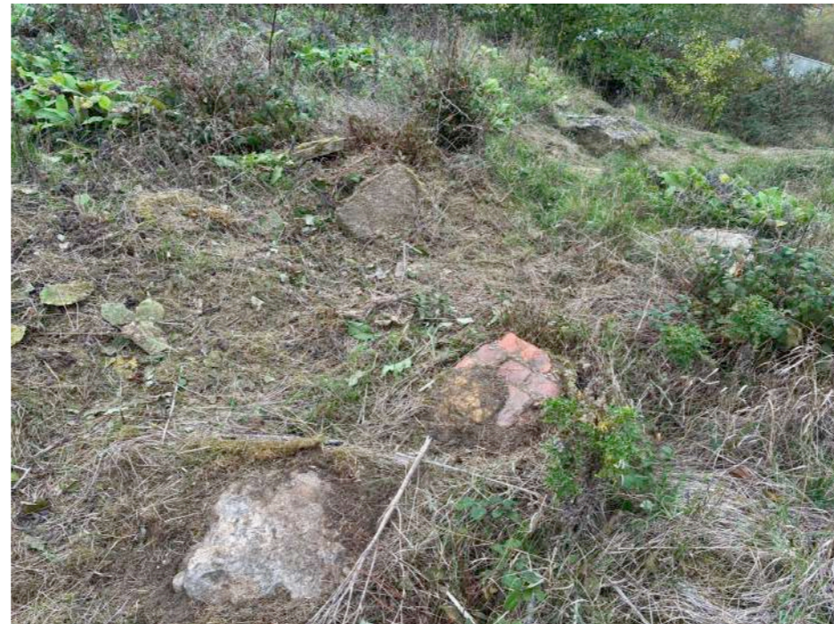
Broken up concrete & brickwork on plateau to the north of the existing building
