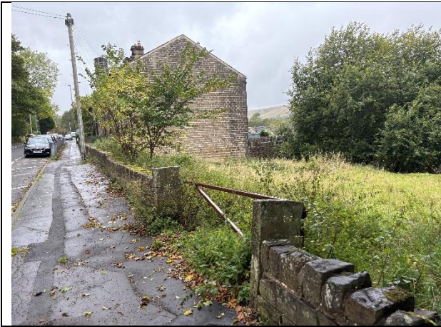
Photo 1: Dry stone wall and tall forbs habitat along the southern boundary.
