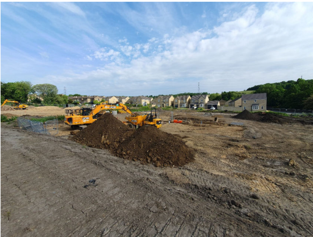
Photograph: 16, Looking north general view across site from the southern boundary, May visit. Topsoil has been stripped and stockpiled on the southern boundary of from which the photo is taken on top of. A stockpile of tree roots mixed in with topsoil in visible in the rear right of the photo. A stock pile of drainage arisings is visible in the foreground on the left.
