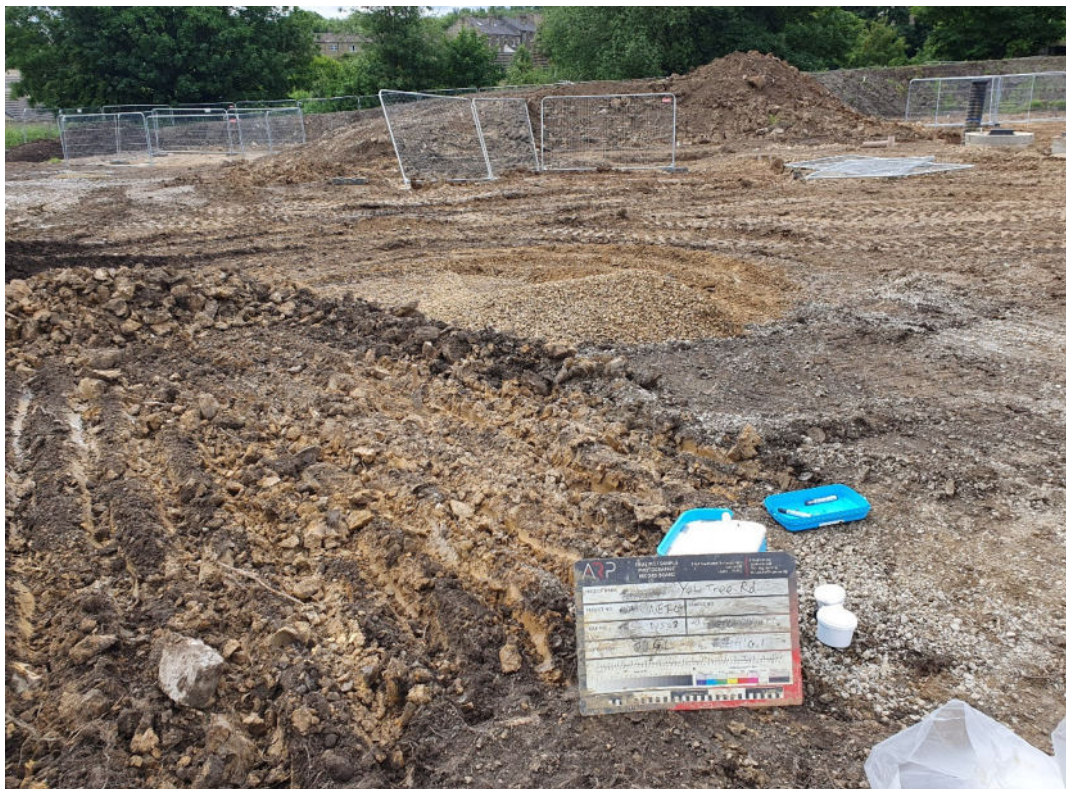
Photograph: 6, Looking south across the area at Location WS08. Area confirmed to have been stripped down to natural clay, June visit. Location of natural subsoil sample taken at locality. Arisings from drainage excavations in back ground.
