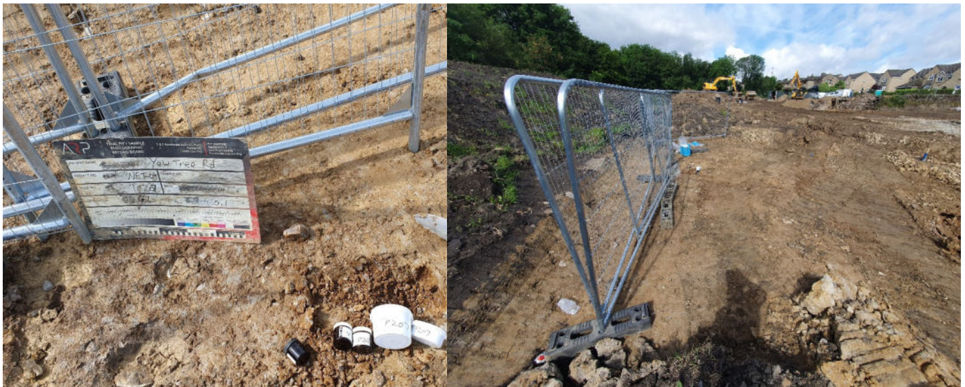
Photograph: 2, Looking west across the 25m 2 excavation area at Location TP207. Area confirmed to have been stripped down to natural clay June visit (Right). Location of natural subsoil sample taken at locality June visit (Left).
