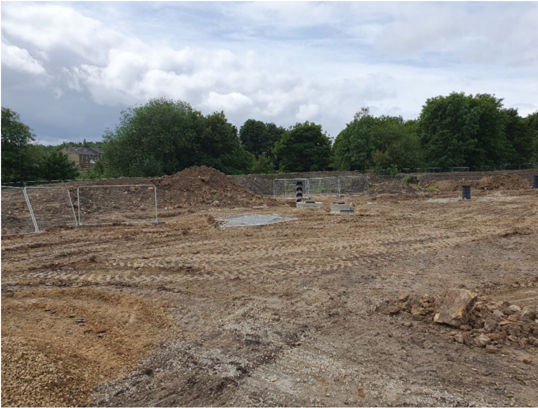
Photograph: 13, Looking south general view across site from the northern boundary, June visit. Topsoil has been stripped and stockpiled on the southern boundary of the site visible along the rear of the photo.
