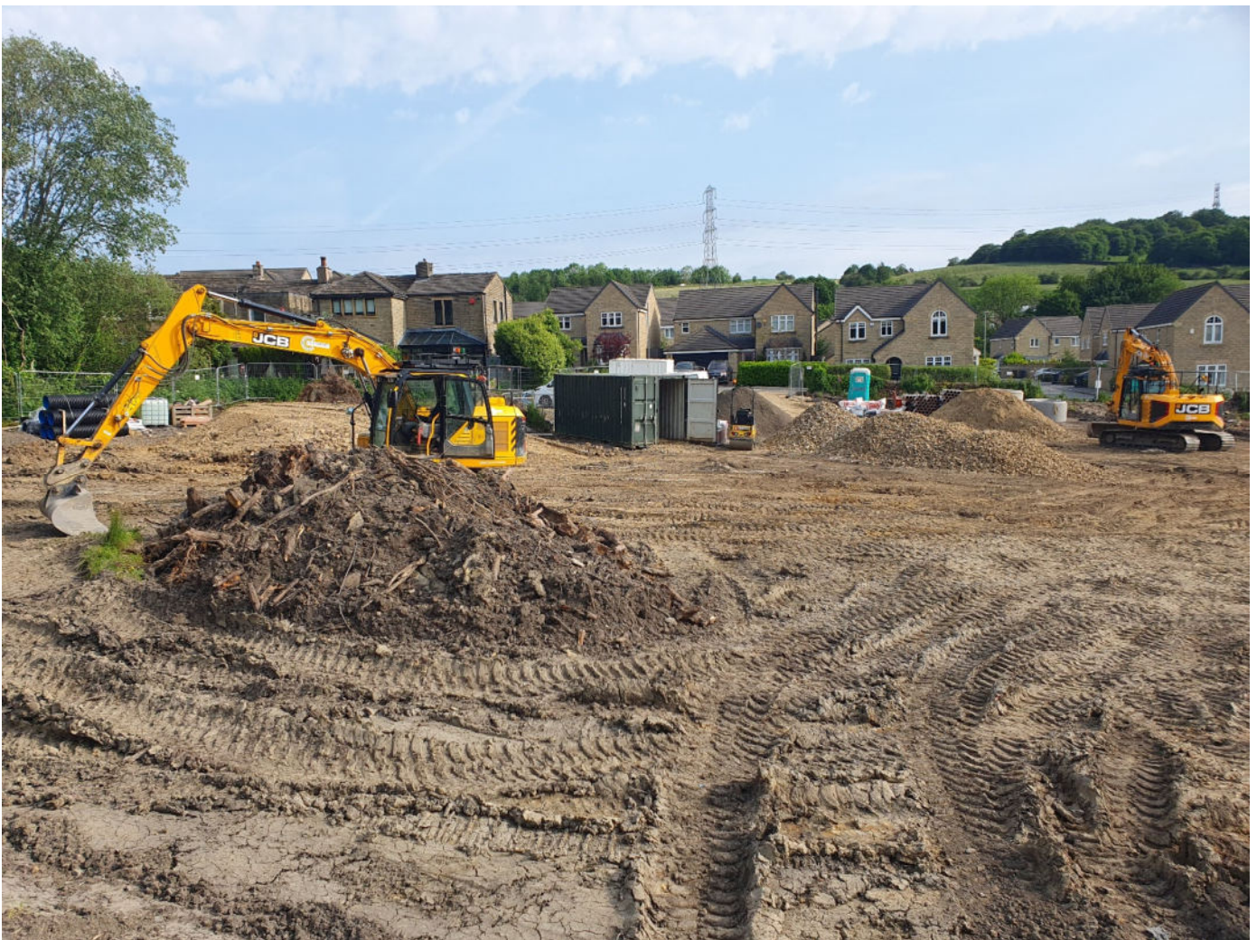
Photograph: 18, Looking north general view across the separate Site A from the southern boundary, May visit. Topsoil has been stripped and stockpiled on the southern boundary of the site. Stockpile of unsuitable tree roots mixed in with topsoil visible at the front of the photo.
