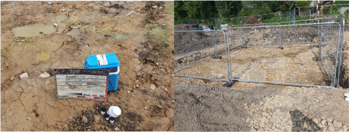
Photograph: 17, Looking west across the 25m 2 excavation area at Location NW Corner, May visit. Area confirmed to have been stripped down to natural clay, May visit (Right). Location of natural subsoil sample taken at locality, June visit.
