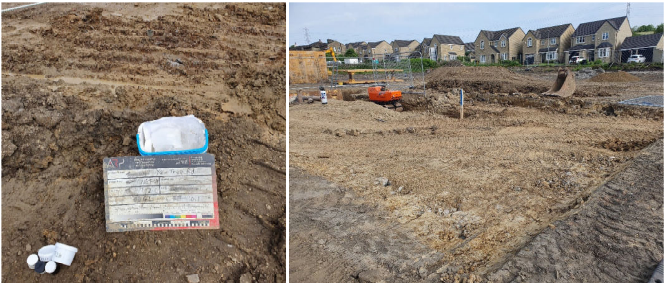
Photograph: 4, Looking northwest across the 25m 2 excavation area at Location TP210. Area confirmed to have been stripped down to natural clay, May visit (Right). Location of natural subsoil sample taken at locality June. Surface had been disturbed by the commencement of works associated with installing site drainage since May visit. (Left).
