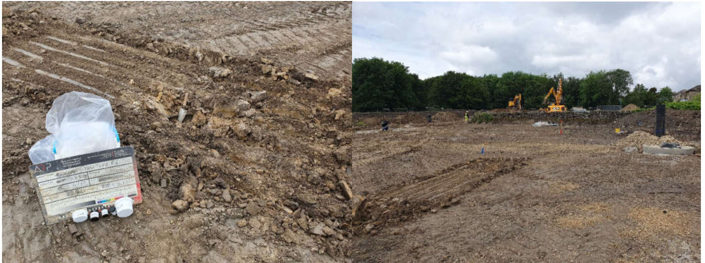
Photograph: 5, Looking southwest across the area at Location WS07. Area confirmed to have been stripped down to natural clay, June visit (Right). Location of natural subsoil sample taken at locality June visit (Left).
