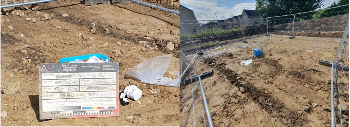
Photograph: 1, Looking southeast across the 25m 2 excavation area at Location TP208. Area confirmed to have been stripped down to natural clay, June visit. (Right). Location of natural subsoil sample taken at locality June visit (Left).
