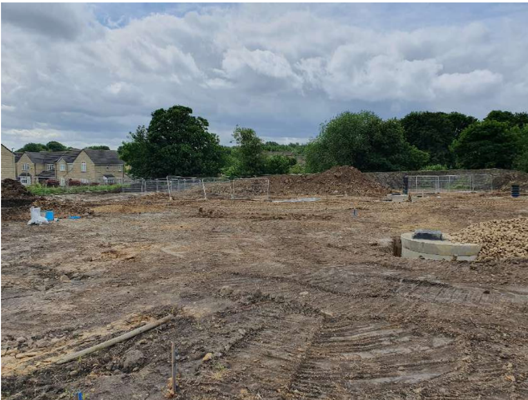
Photograph: 14, Looking south general view across site from the northern boundary, June visit. Topsoil has been stripped and stockpiled on the southern boundary of the site visible along the rear of the photo.
