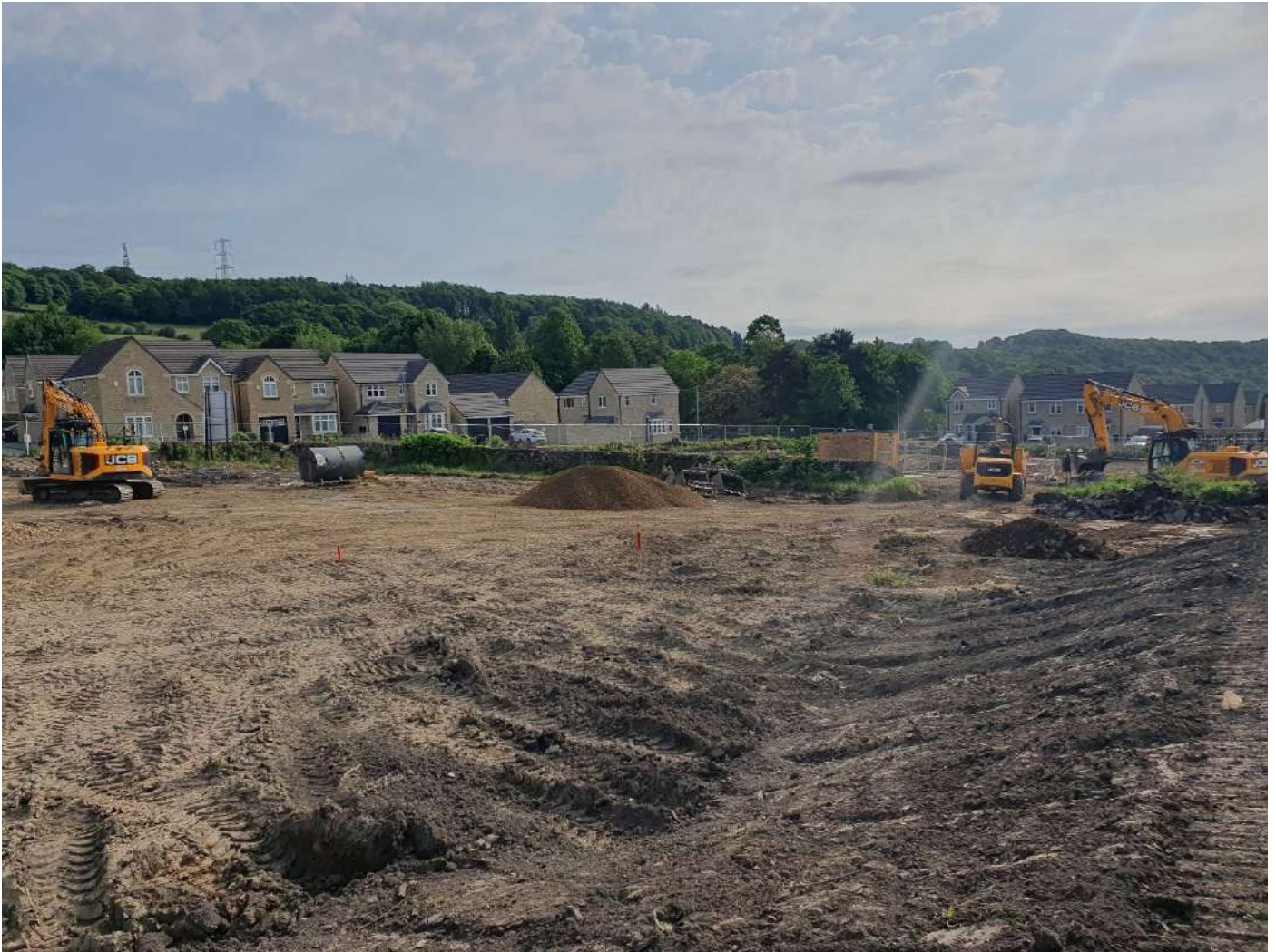
Photograph: 19, Looking northeast general view across the separate Site A from the southern boundary, May visit. Topsoil has been stripped and stockpiled on the southern boundary of the site visible in the foreground.
