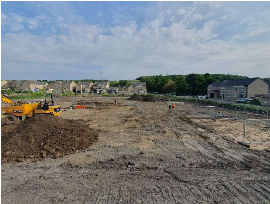
Photograph: 15, Looking north general view across site from the southern boundary, May visit. Topsoil has been stripped and stockpiled on the southern boundary of from which the photo is taken on top of. A stockpile of unsuitable tree roots and topsoil in visible in the rear right of the photo. A stock pile of drainage arisings is visible in the foreground on the left.
