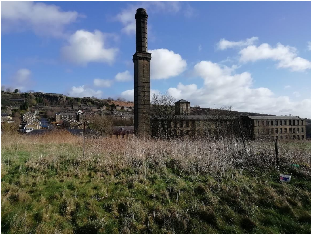
Figure 10: View looking northeast across the site towards the converted Mill.
