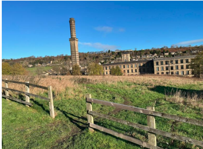
Figure 9 View across the site showing change in levels towards the mill complex
