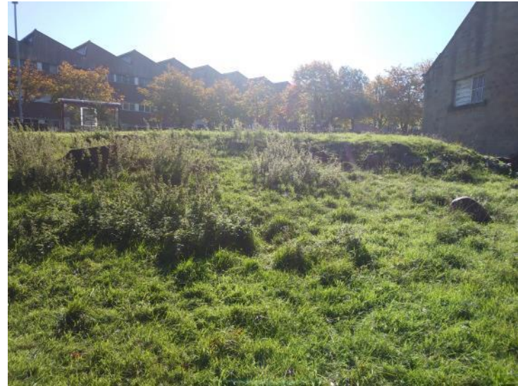
Photograph 10 – Retained earth behind small wall structure
