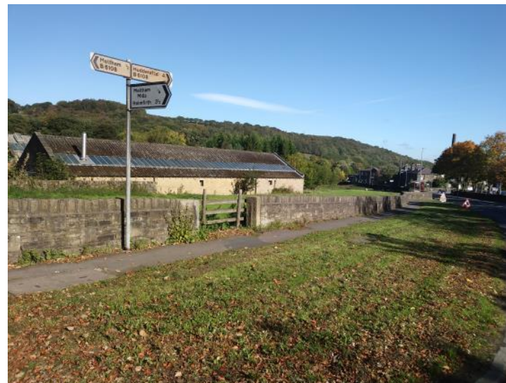
Photograph 2 – View north along the site boundary with Huddersfield Road
