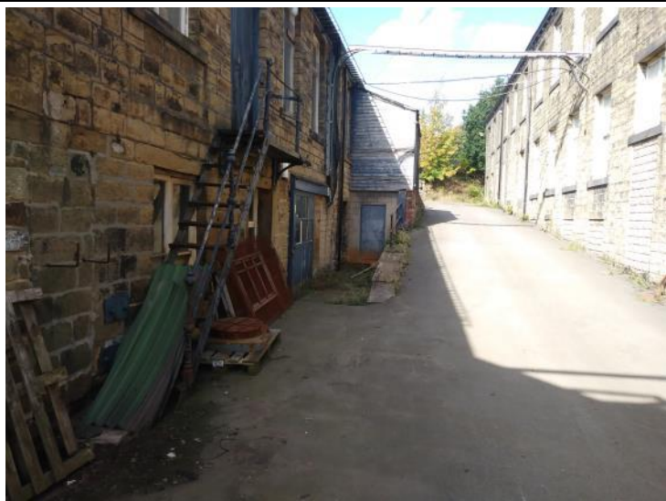
Photograph 59 – View north-west toward retaining wall
