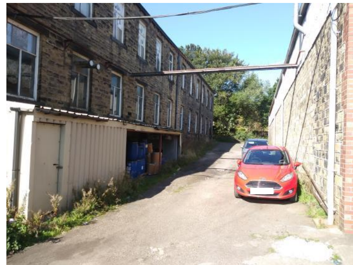
Photograph 46 – Unbunded chemical storage area in Spinksmire Mill
