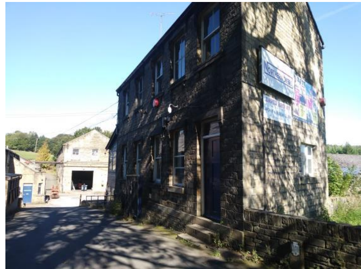
Photograph 12 – Northern Dyers building near site entrance
