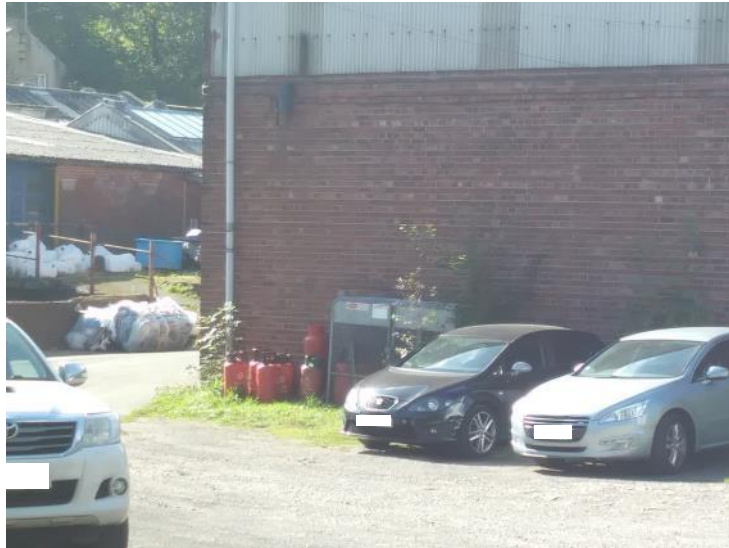
Photograph 41 – Unbunded gas bottle storage area at north-eastern edge of Mill
