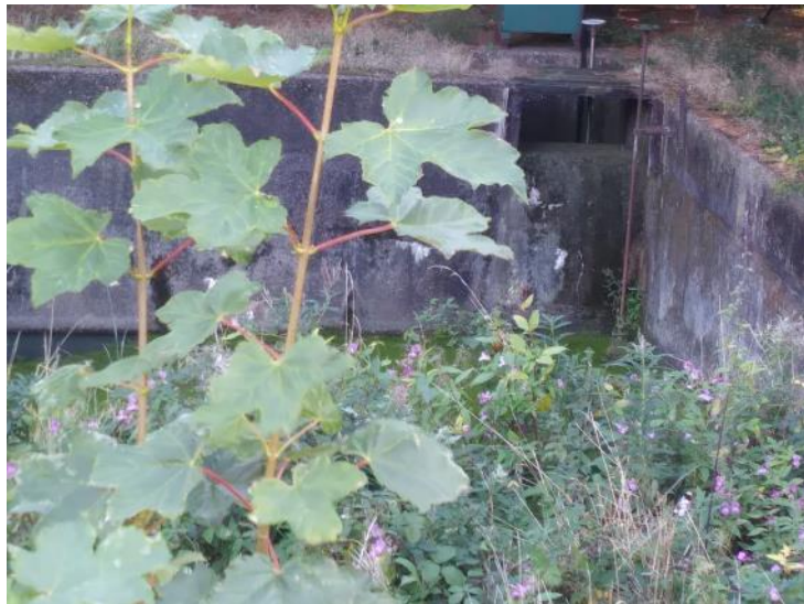
Photograph 43 – Open concrete water storage tanks within south of wooded area
