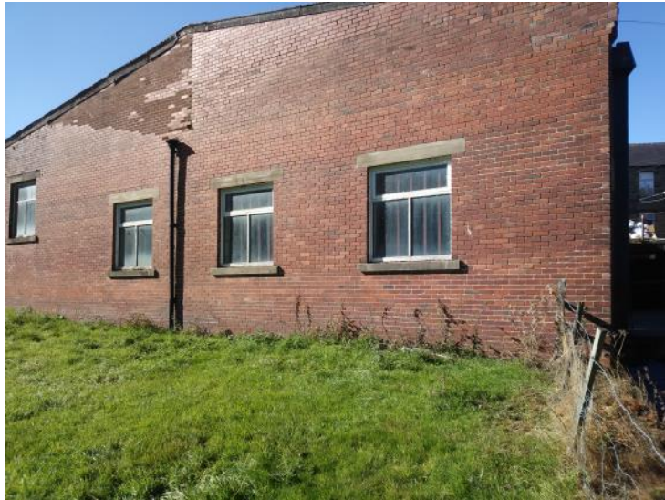
Photograph 9 – Brick built warehouse/workshop with possible asbestos roofing
