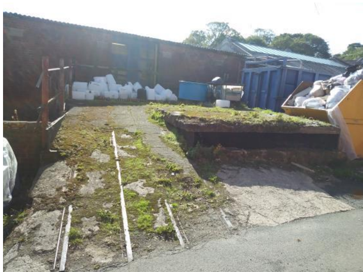
Photograph 45 – Raised waste storage area above Meltham Dike culvert (exit)
