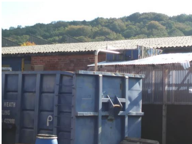
Photograph 55 – Asbestos sheet roofing on warehouse closest to Huddersfield Road
