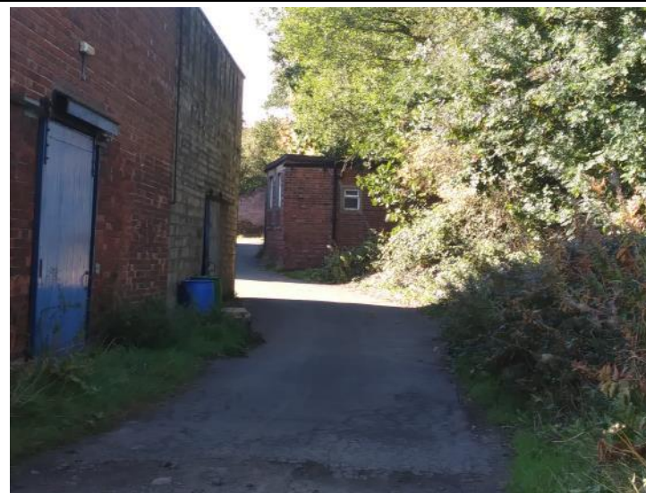
Photograph 36 – View along north-western edge of Spinksmire Mill
