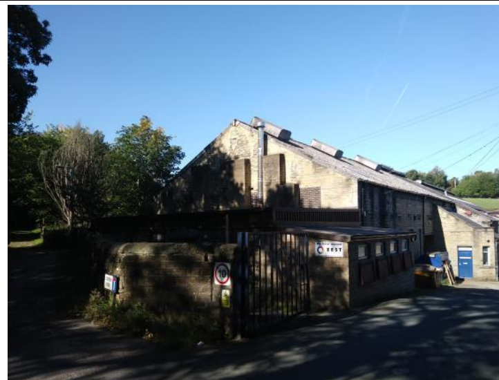
Photograph 14 – Brick built warehouse/factory with possible asbestos roofing
