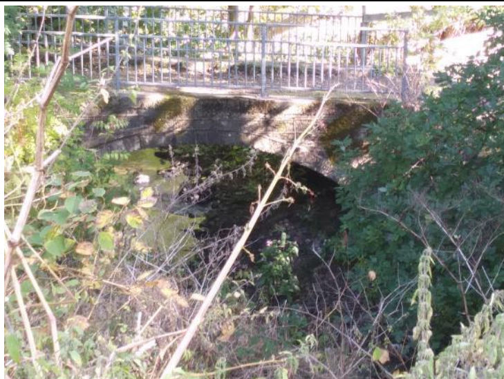
Photograph 39 – Bridge enabling vehicular access to track from Huddersfield Road
