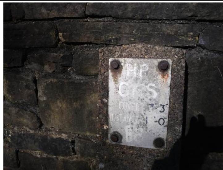
Photograph 4 – High pressure gas marker adjacent to site entrance
