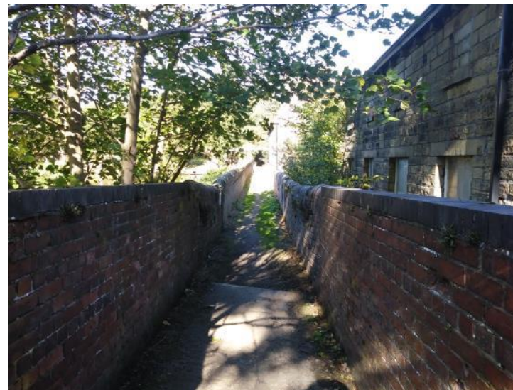
Photograph 18 – Wall lined public footpath
