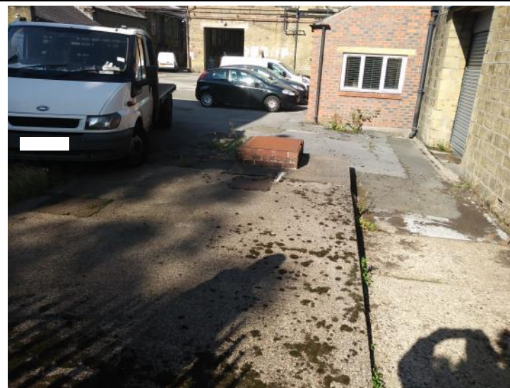
Photograph 64 – Interceptor drain north of Northern Dyers building
