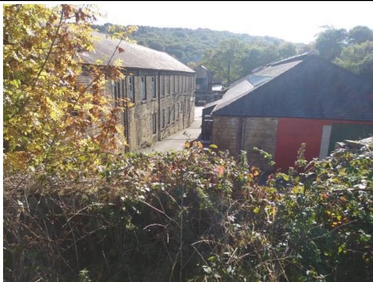
Photograph 35 – View of Spinksmire Mill warehouses from raised grazing field
