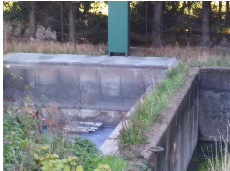
Photograph 42 – Open concrete water storage tanks within south of wooded area
