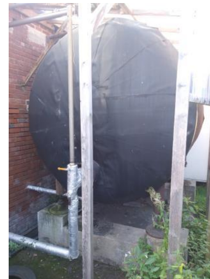
Photograph 56 – Fuel storage tank above Meltham Dike culvert
