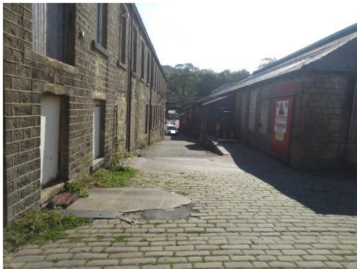
Photograph 53 – View south-east toward site entrance from retaining wall
