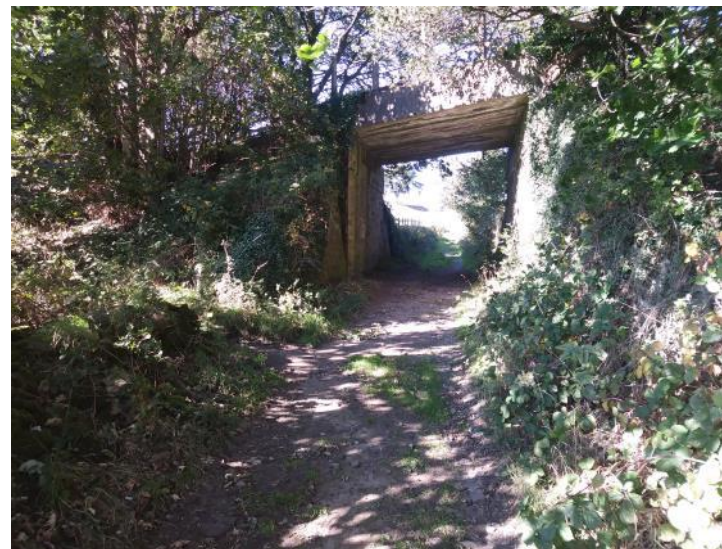
Photograph 30 – Track passageway beneath former railway line
