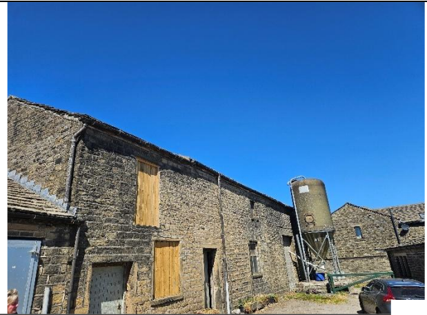
Photo 20: Eastern facing wall of building 4.
