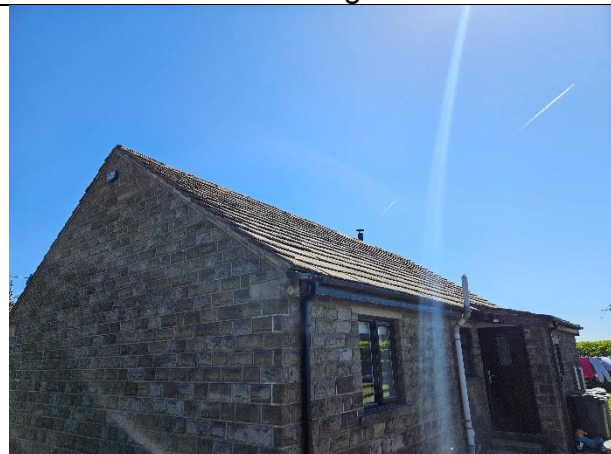
Photo 5: Northern facing view of building 6.
