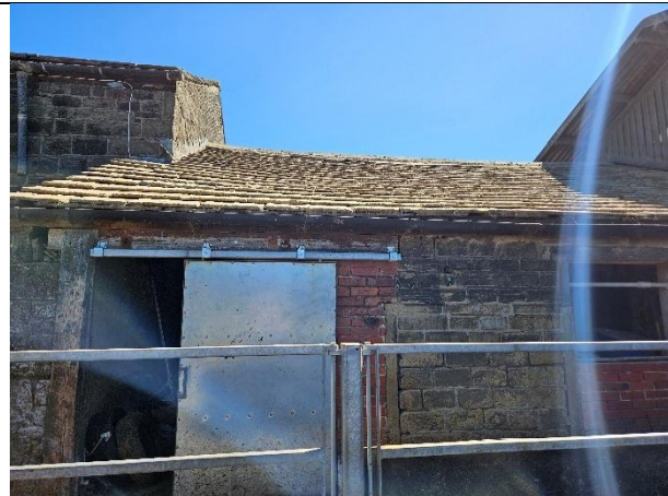
Photo 17: Western facing view of building 4
