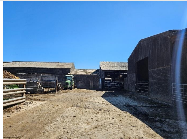
Photo 15: Access to buildings 2, 3 and 4.
