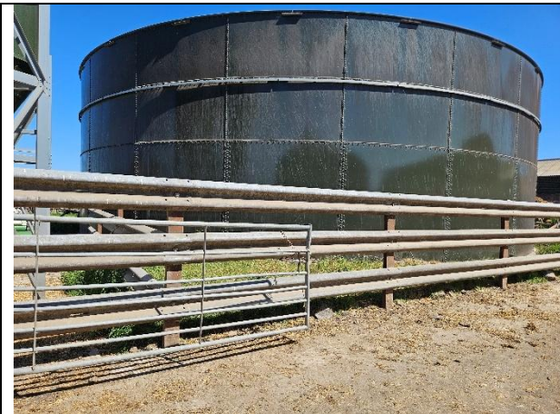
Photo 13: Cylindrical structure in the north of the site.
