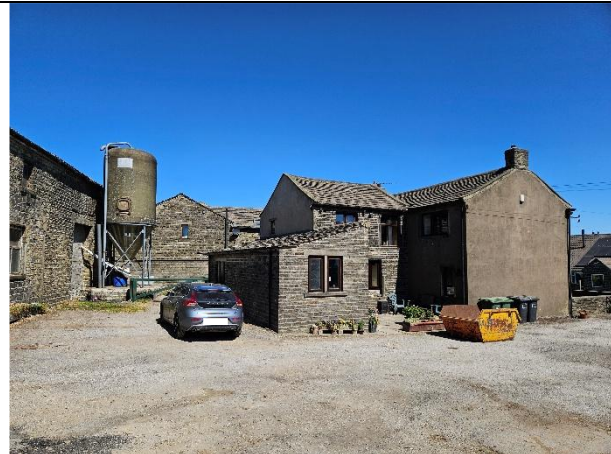
Photo 7: Western facing view of building 7.
