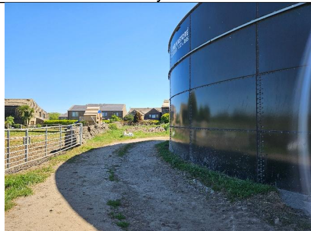
Photo 11: Developed land sealed surface and grassland to the north of the metal cylindrical structure.
