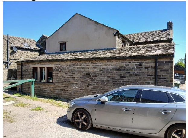
Photo 34: Southern facing wall of building 6.
