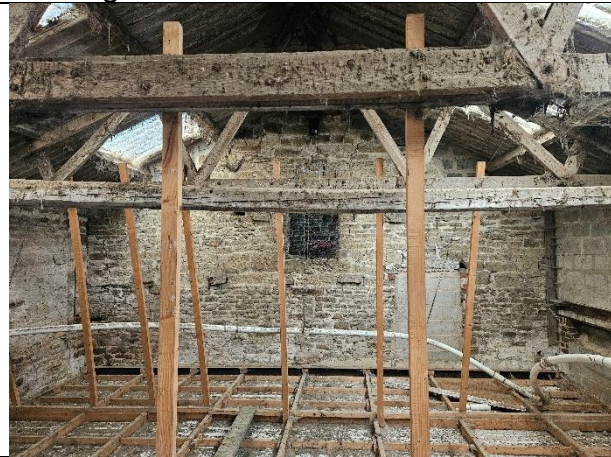
Photo 27: Second story view of building 4.
