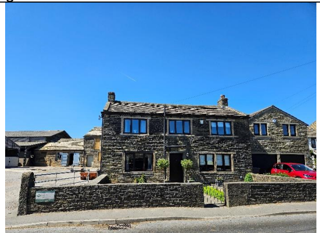
Photo 4: Eastern facing view of building 7.
