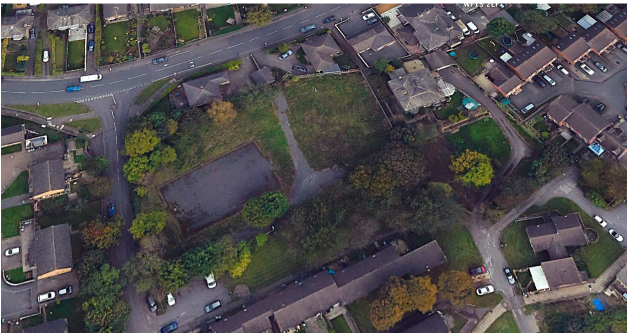
Figure 3. Current aerial view, dated 3 September 2023. Former Arena building demolished and MUGA pitched derelict
