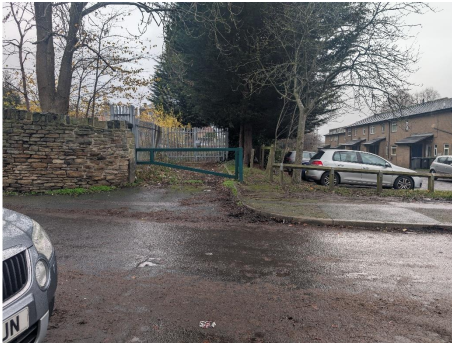
Photo 1: Existing Access Junction
