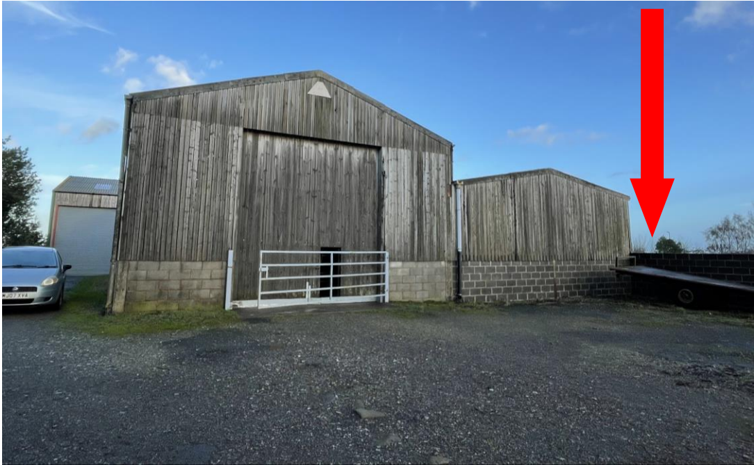
The three existing farm buildings at the Birdsedge Farmyard. The new building will attach to the building on the RHS of the photograph
