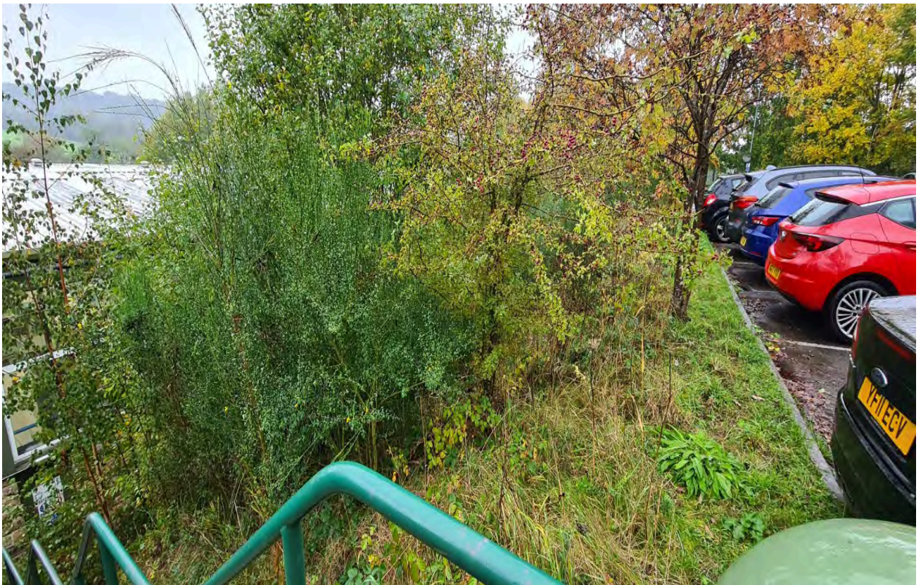
Photograph 6 – Steeply sloping bank in eastern site area between car park and main building.
