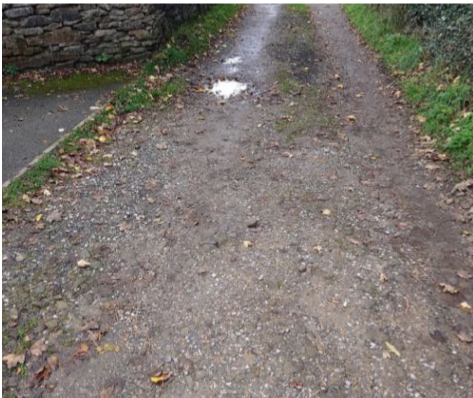
Figure 76 Dam Head location BS
