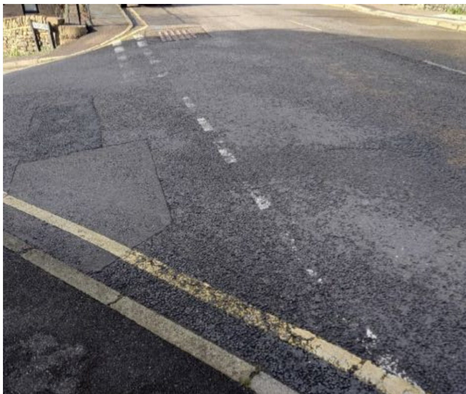
Figure 2 Co-op Lane location A
