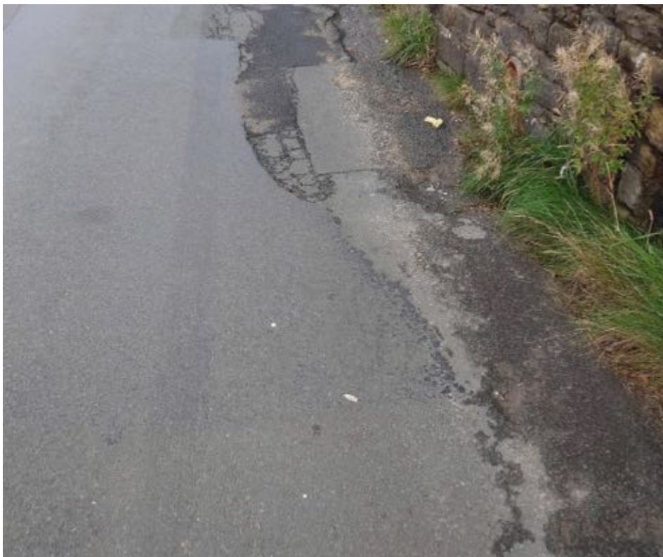
Figure 64 Dobb Lane location BH
