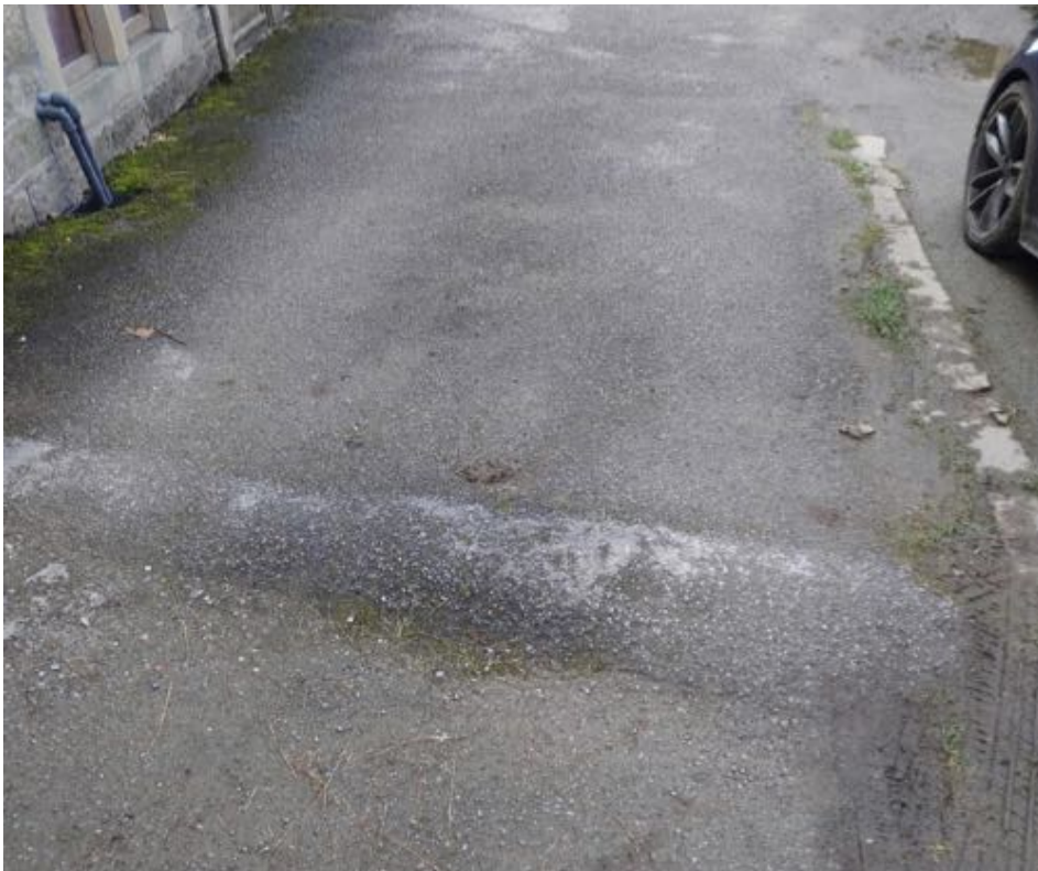
Figure 79 Dam Head location BV
