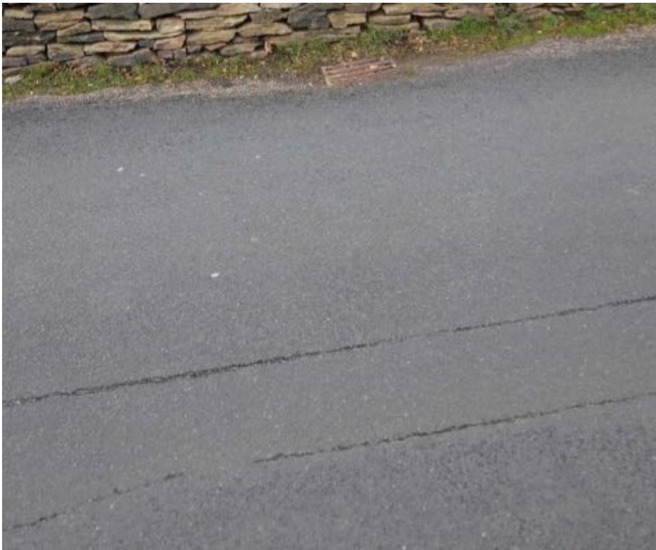
Figure 62 Dobb Lane location BF
