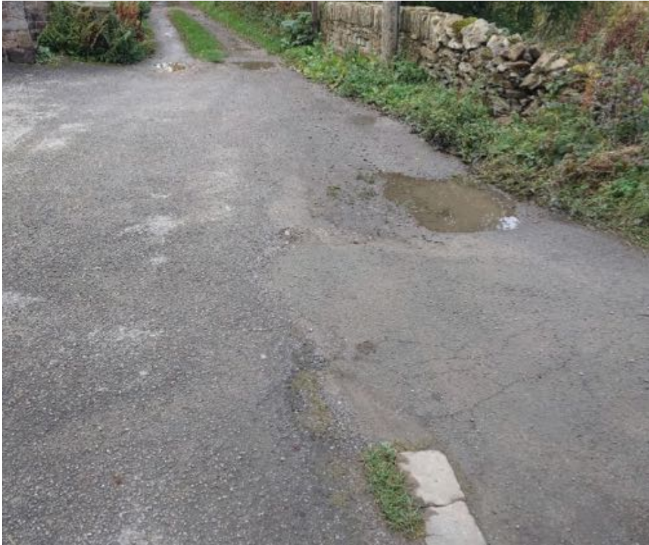
Figure 78 Dam Head location BU
