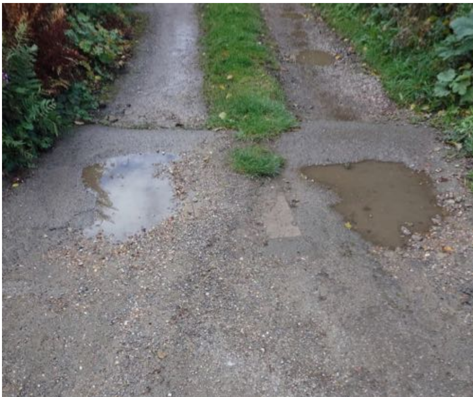
Figure 77 Dam Head location BT
