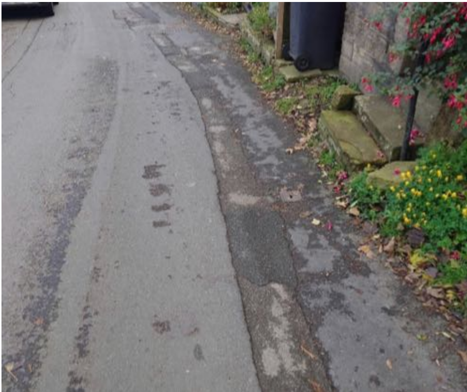
Figure 44 Dobb Lane location AN
