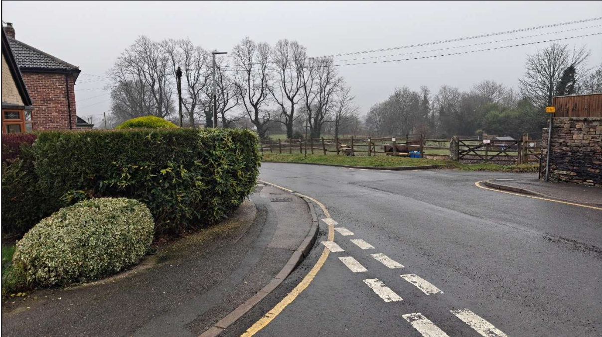
Left visibility splay from 2.4m setback at Woodward Court junction with Wellhouse Lane
