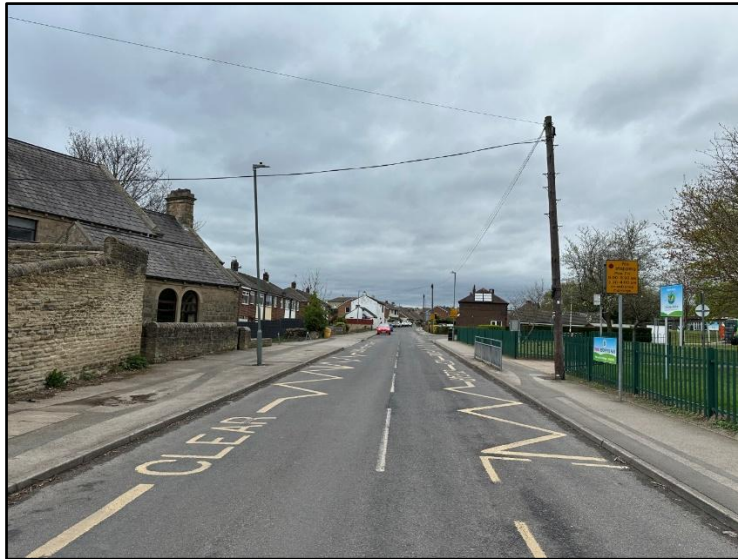
Image 2.6 School Keep Clear Marking – Wellhouse Lane
