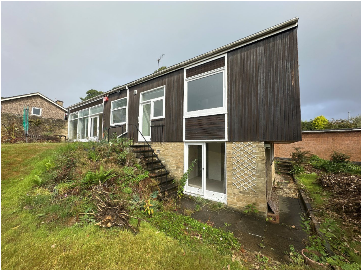
Above: Existing rear of building
