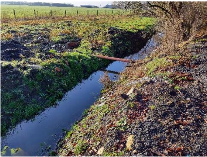
Figure 15 Typical view of drainage ditch.
