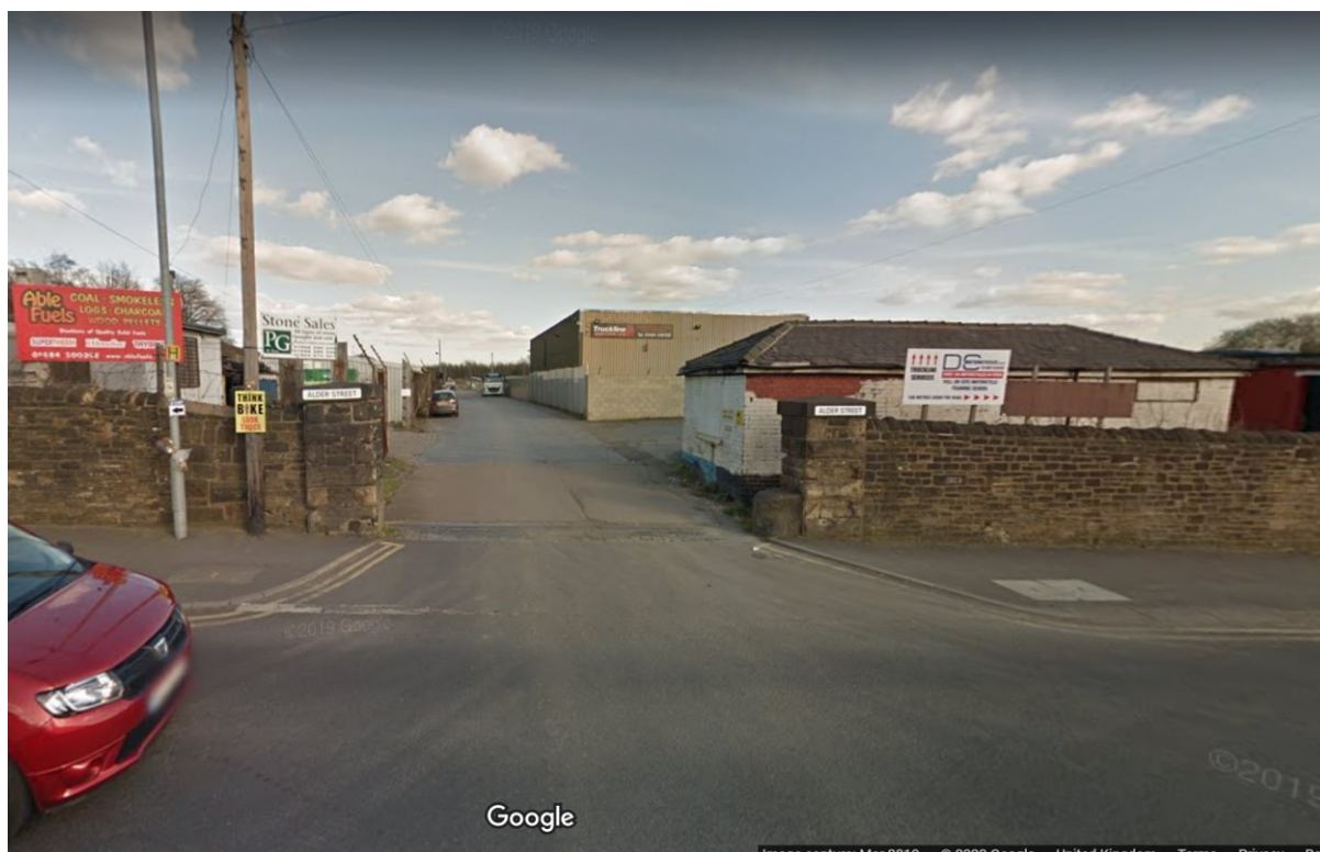
Insert 3-1 Existing Site entrance to be retained during enabling works
