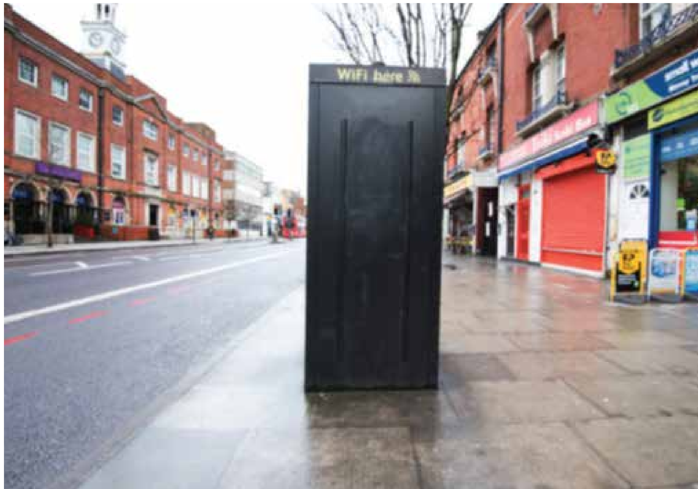
Existing Telephone kiosk
