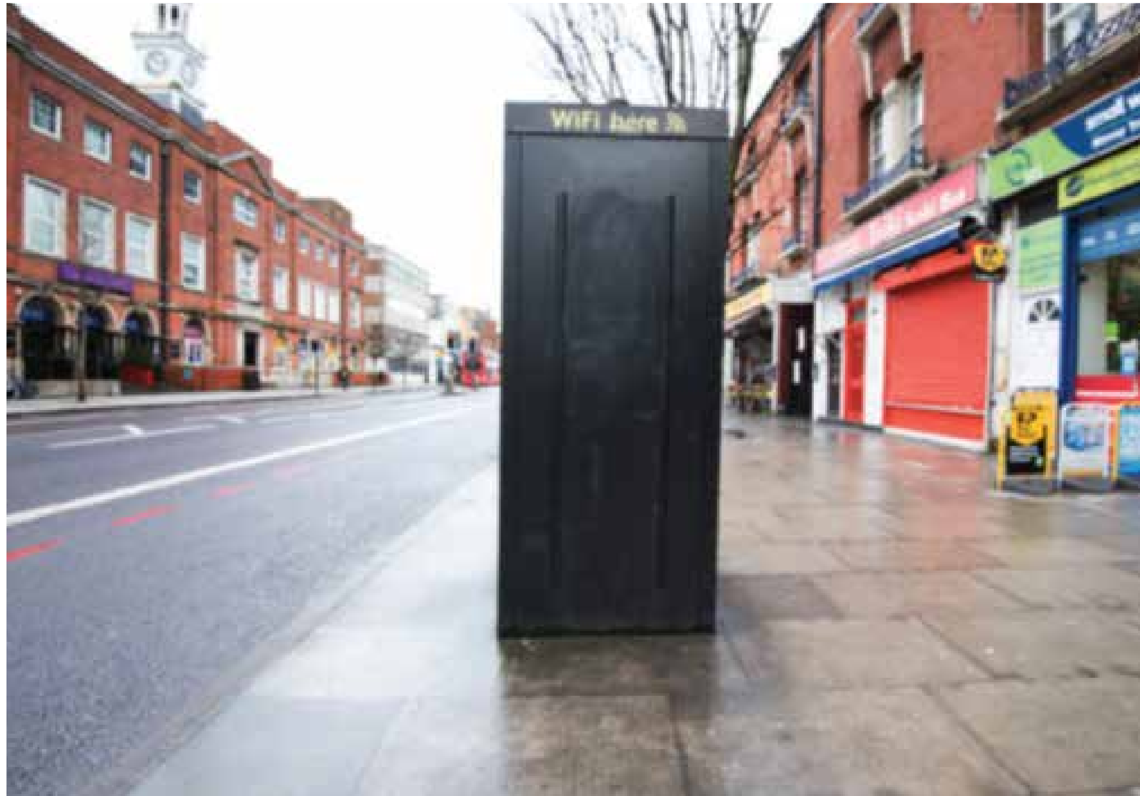
Existing Telephone kiosk
