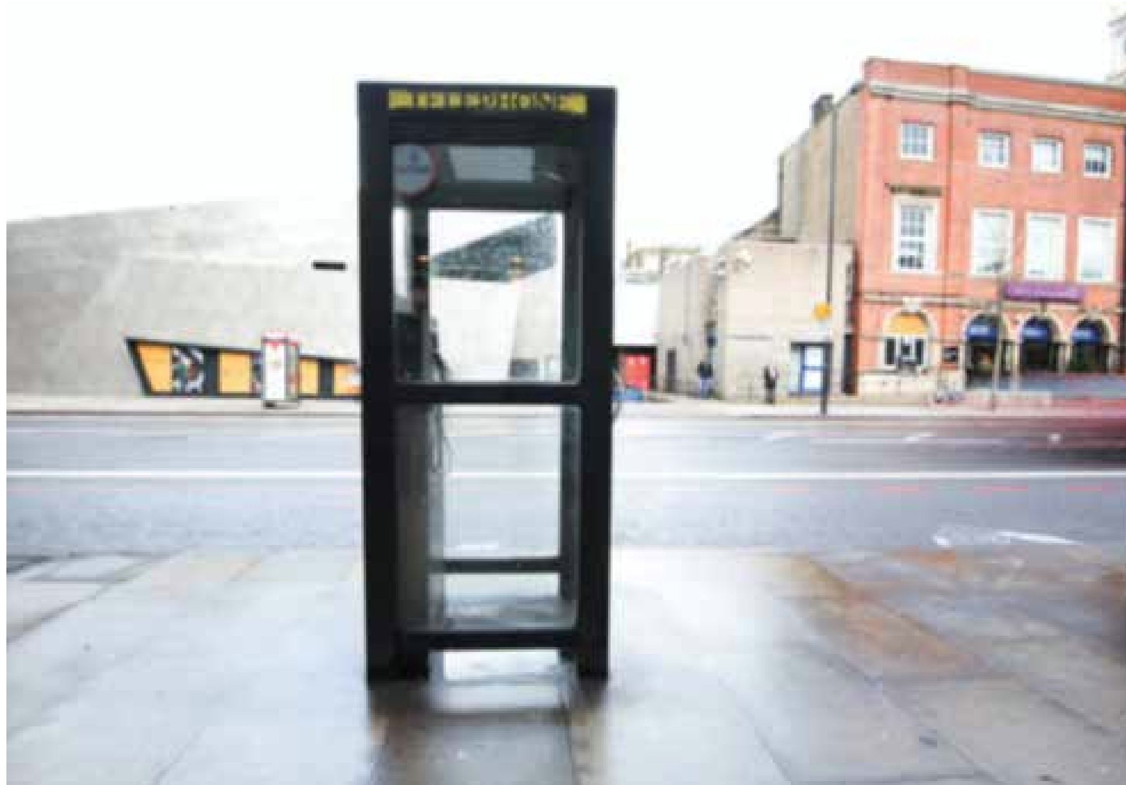
Existing Telephone kiosk
