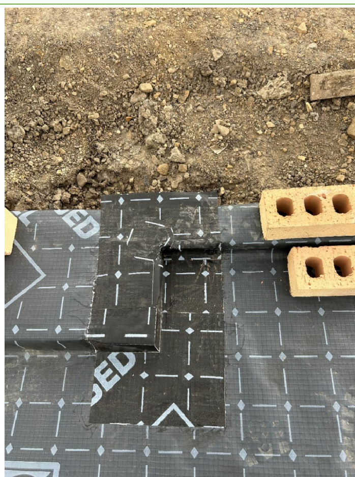
Examples of taped corners – Plots 553-554
