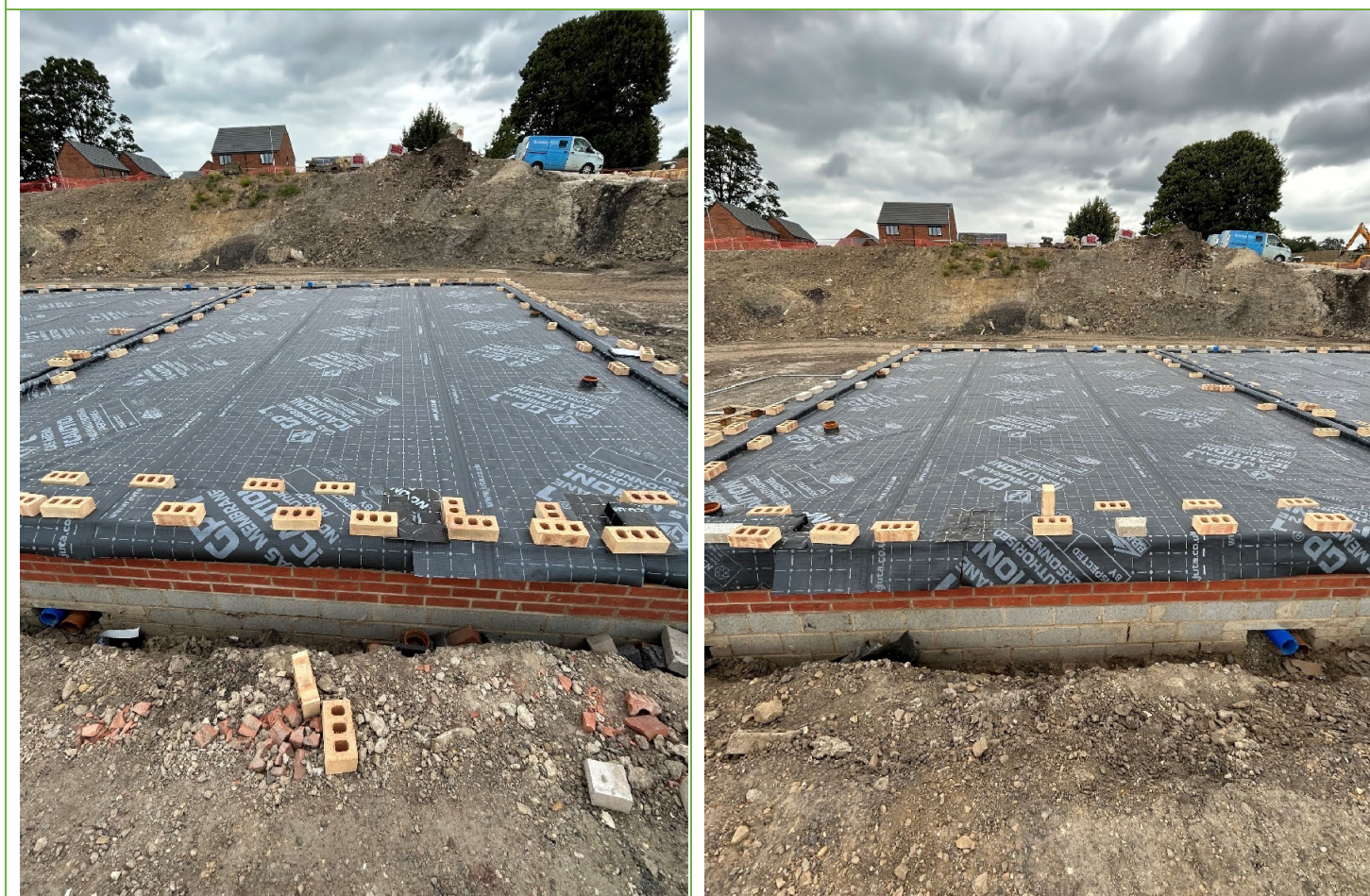
Example of Membrane across floor – Plots 553-554
