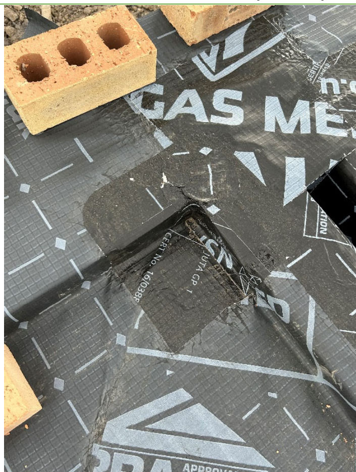
Examples of taped corners – Plots 553-554
