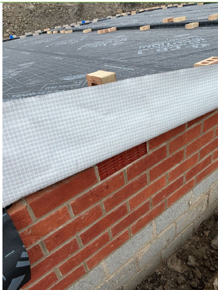
Examples of telescopic vents – Plots 553-554
