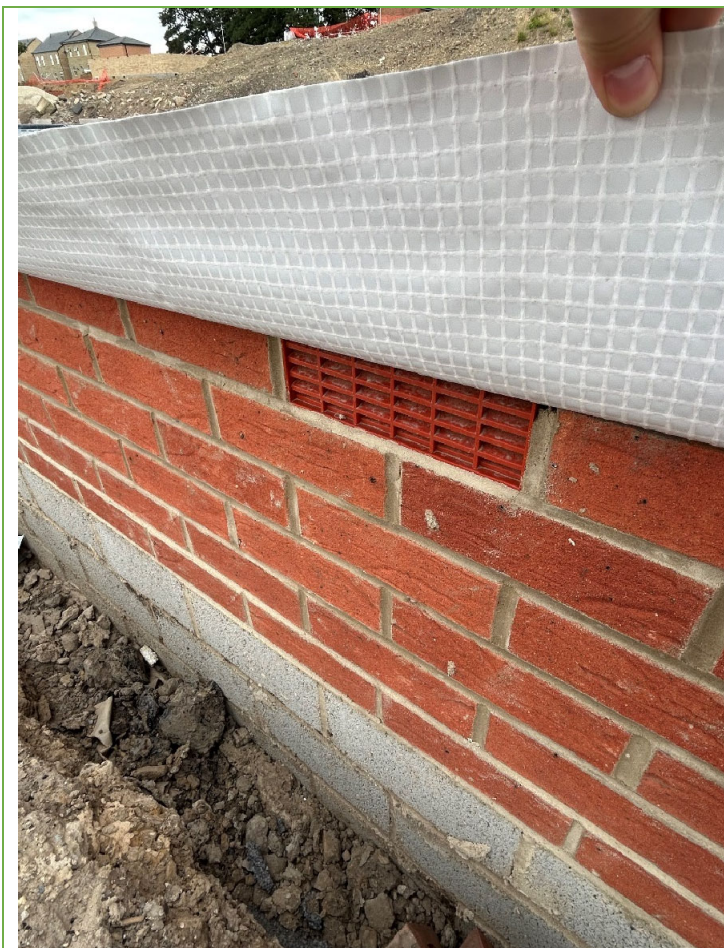
Examples of telescopic vents – Plots 553-554
