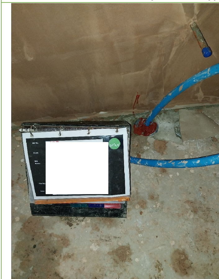
Example of the closed cell foam placed around the water annulus – Plots 553-554
