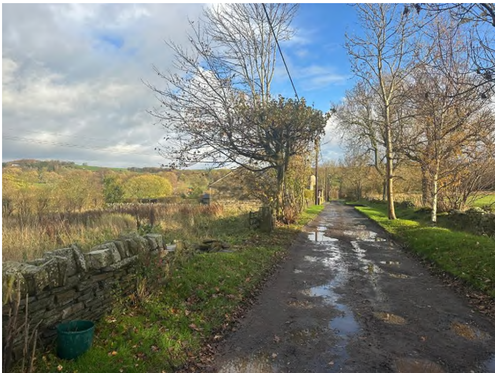
3. The condition of the lane. This was taken last year when the initial planning application was submitted. The conditions have worsened since and holes are deeper.
