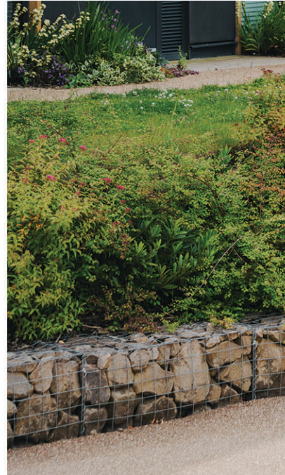
retaining wall (gabion) ornamental planting
