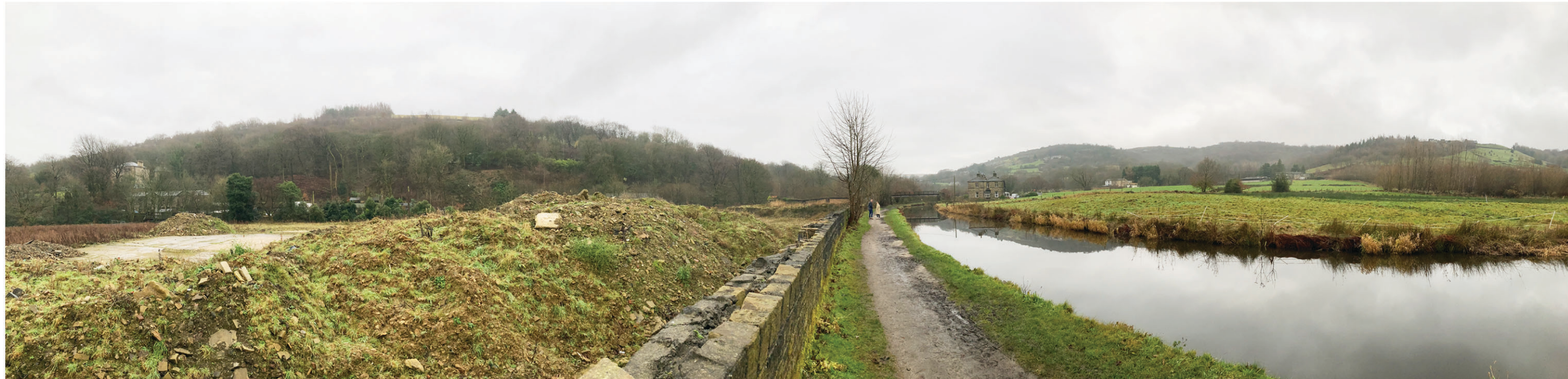
site - towpath - canal
