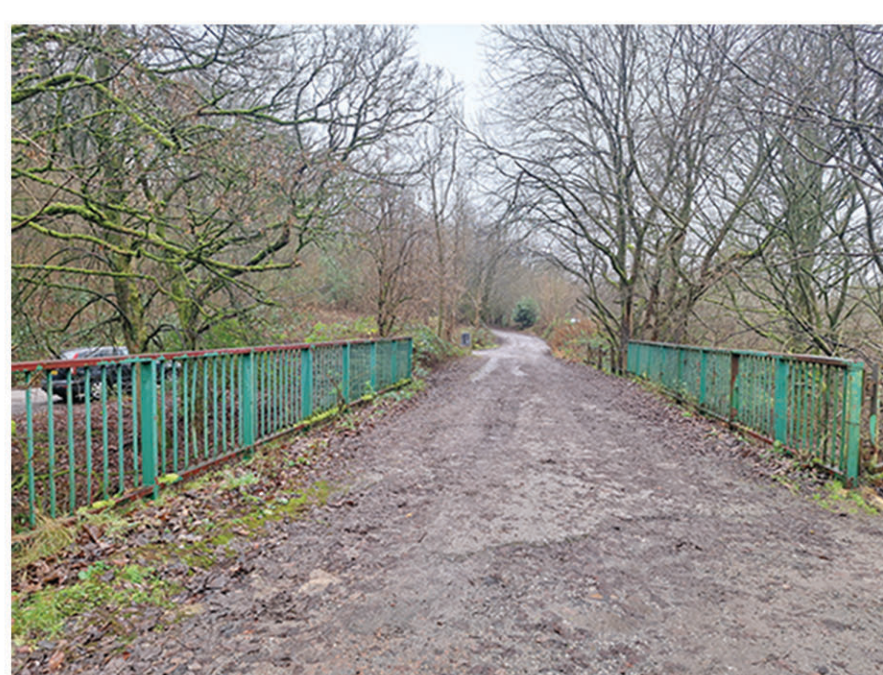
access road bridge
