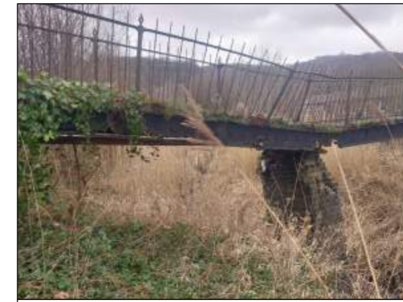
Photo 8 Evidence of former footbridge (now in disrepair), located over infilled mill pond.
