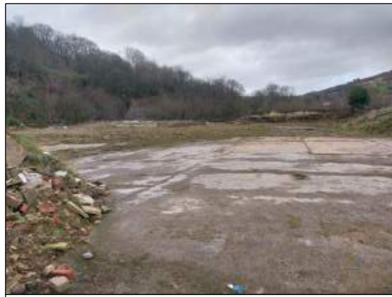
Photo 4 View of remnant concrete slab, associated with former mill, with demolition rubble stockpiles.
