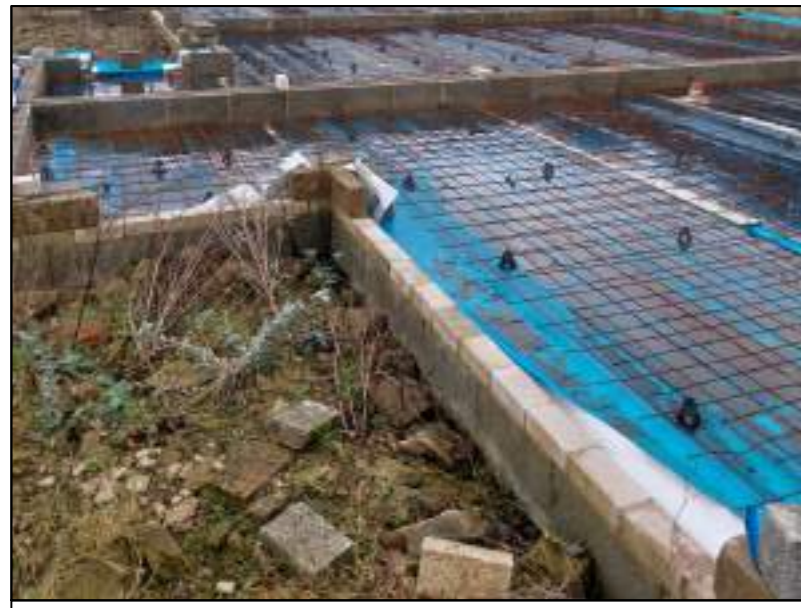
Photo 3 View of former, abandoned residential development, undertaken by previous developer.
