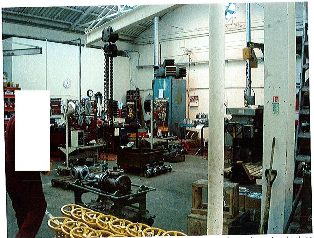
Storage area for equipment and valves
