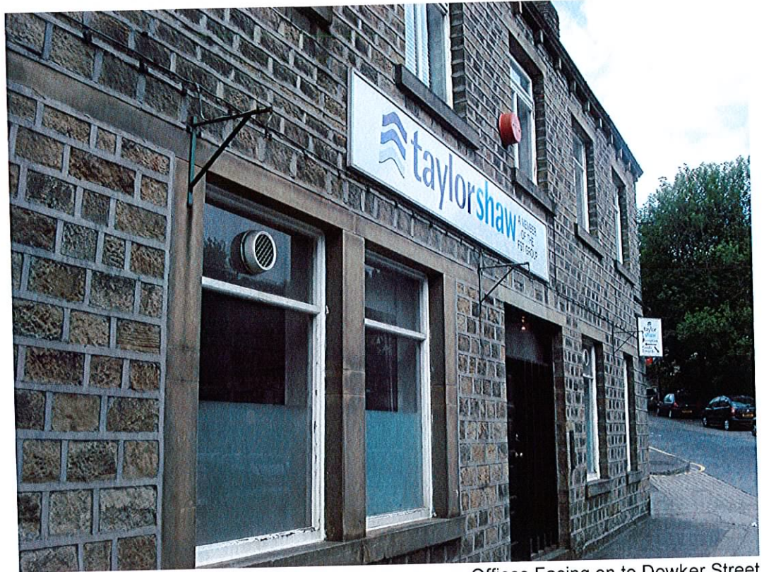
Offices Facing on to Dowker Street
