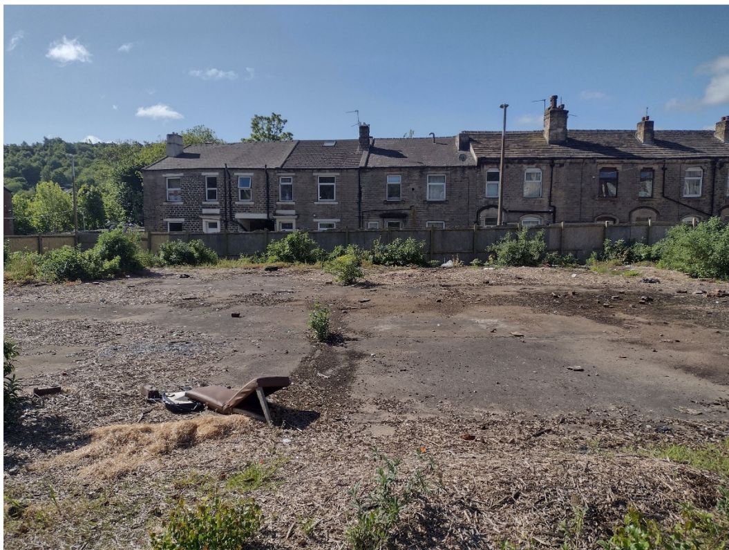
Photograph 8: Concrete floor slab at the southern end of the site, facing south.
