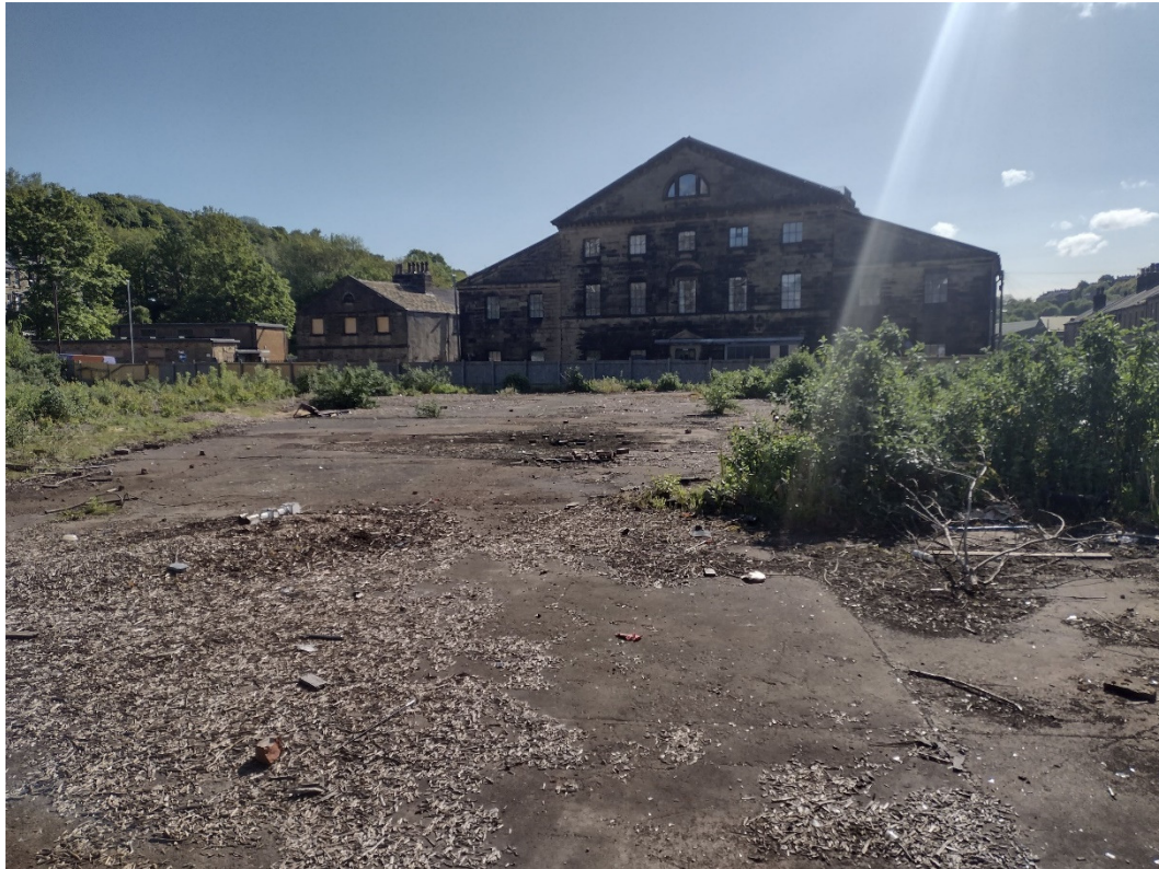
Photograph 9: Concrete floor slab at the southern end of the site, facing east.
