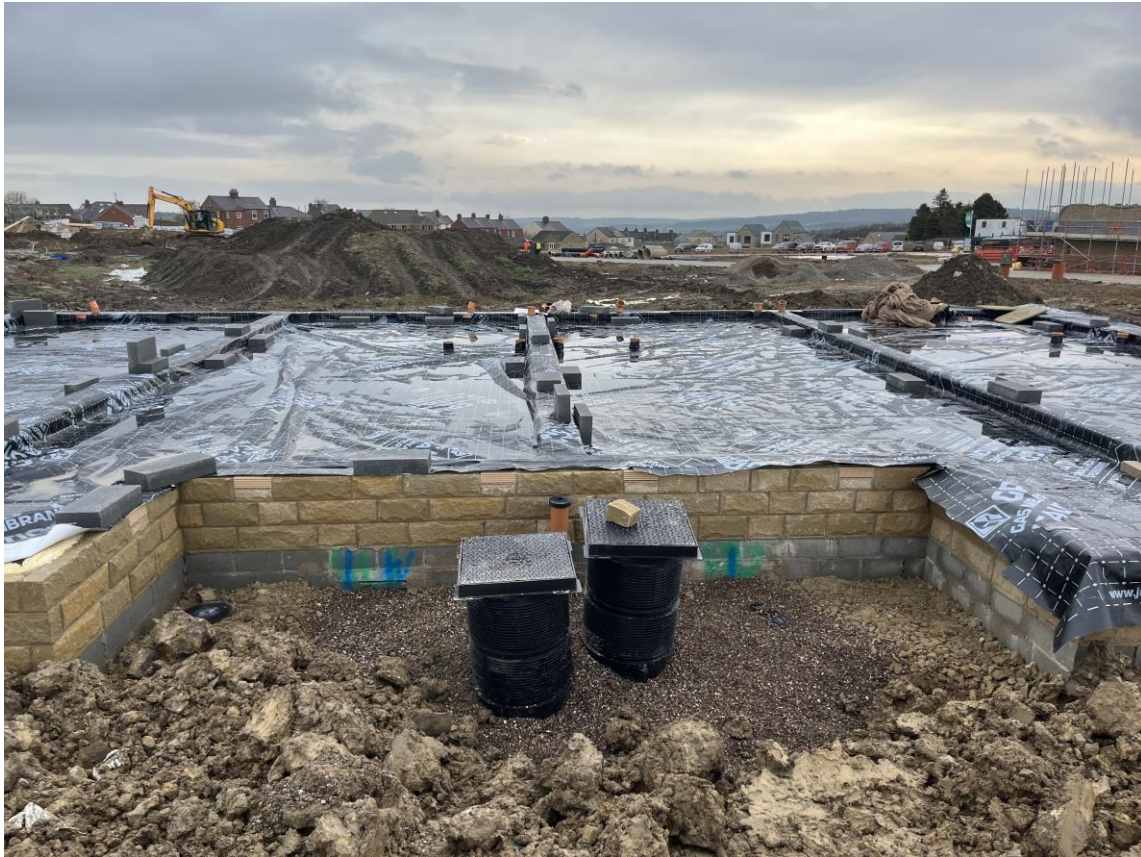
Plots 75-78 – Internal wall membrane layout with welds
