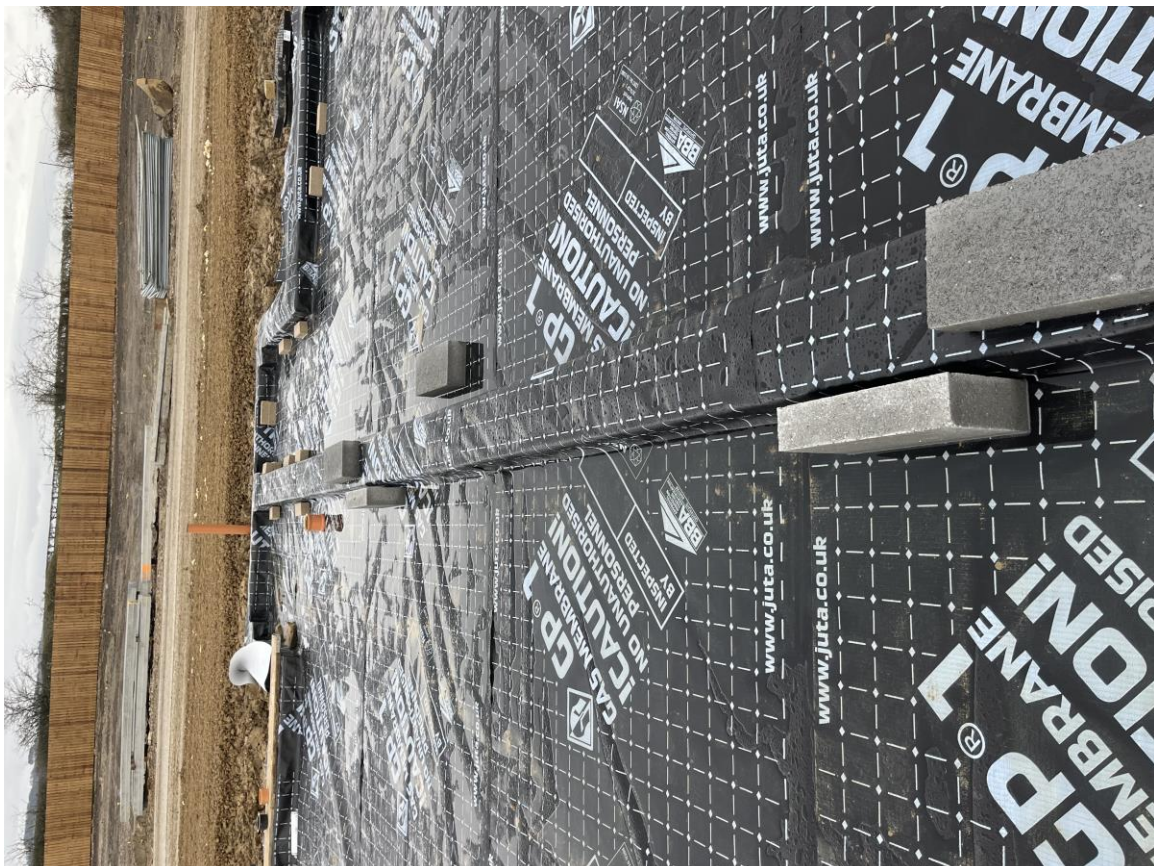
Plots 75-78 – Internal wall membrane layout with welds
