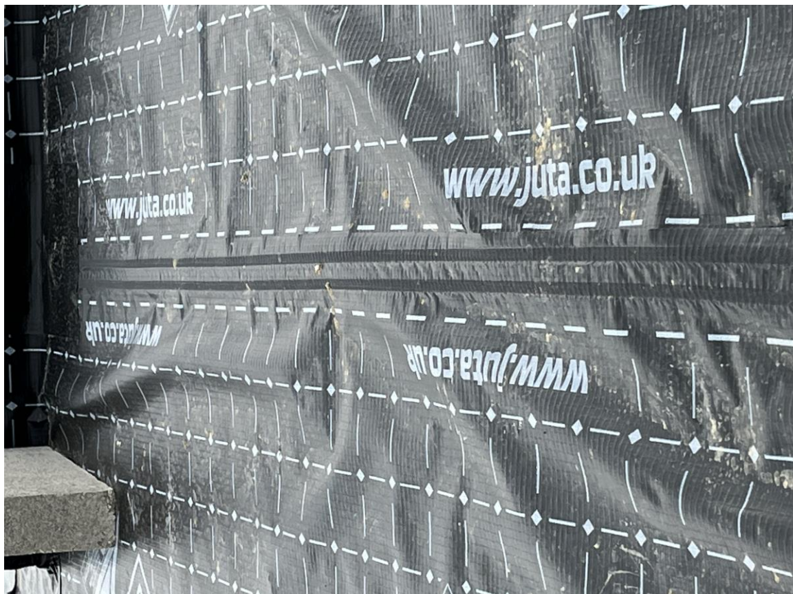
Plot 52 – Membrane layout with weld joint
