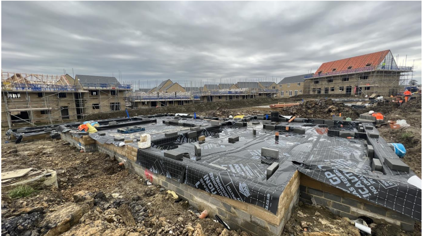
Plot 71 – Membrane layout with tophats and jointing
