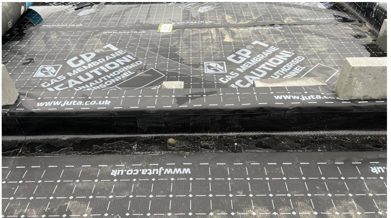
Plots 97 & 98 – Membrane layout with internal wall and jointing
