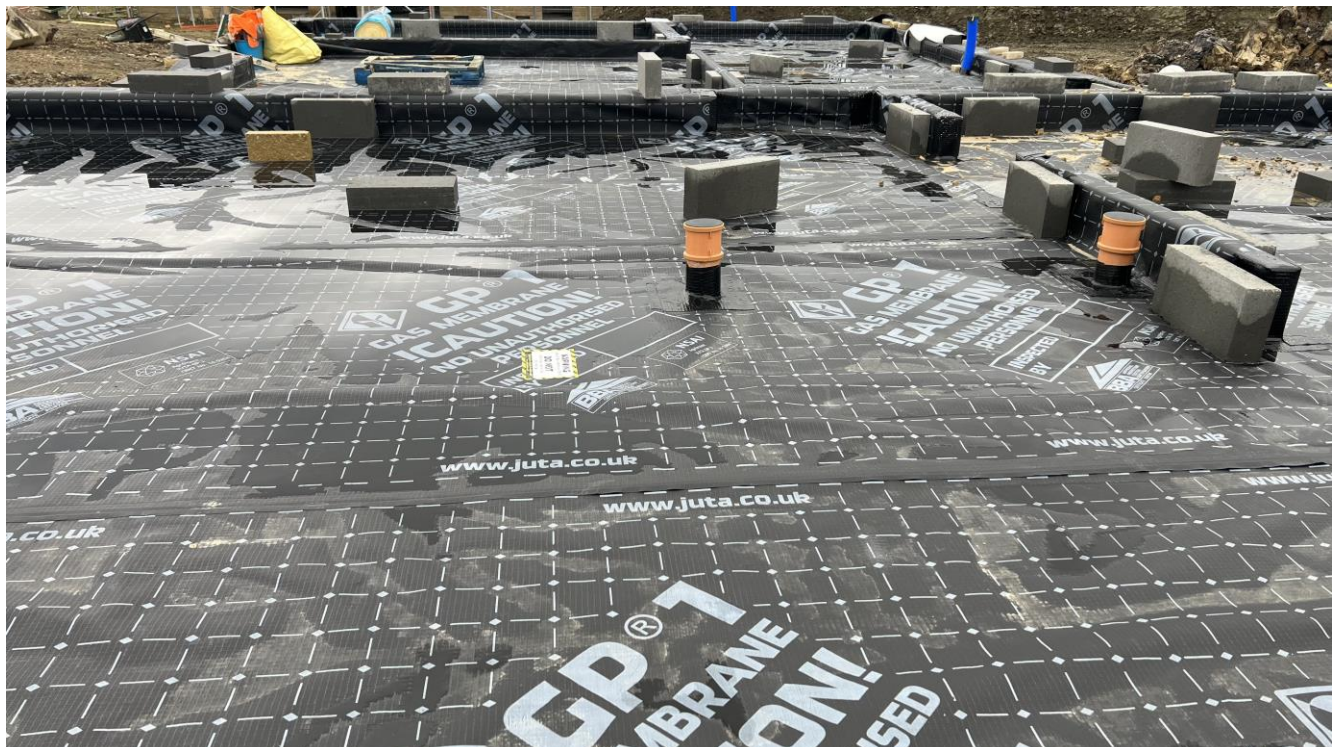
Plot 70 - Membrane layout with tophats and jointing
