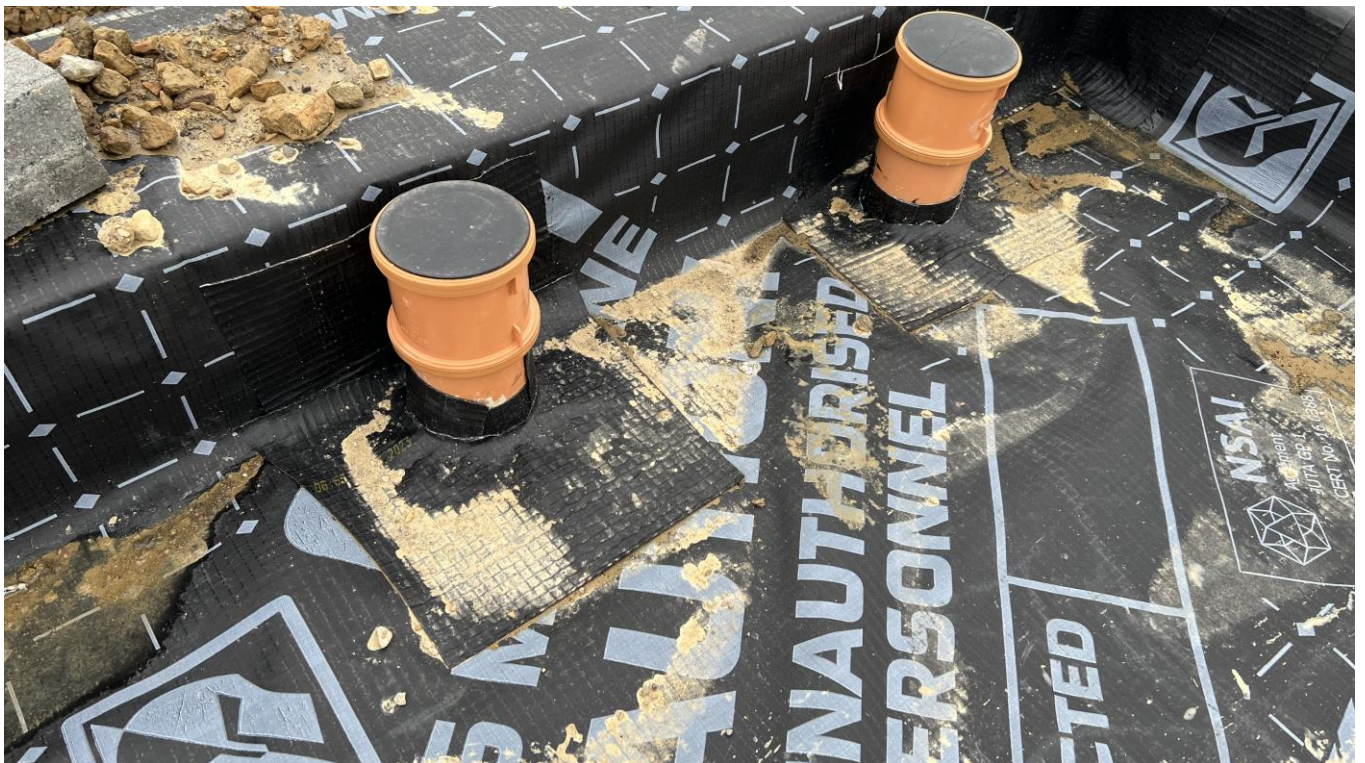
Plot 71 – Membrane layout with tophats and jointing
