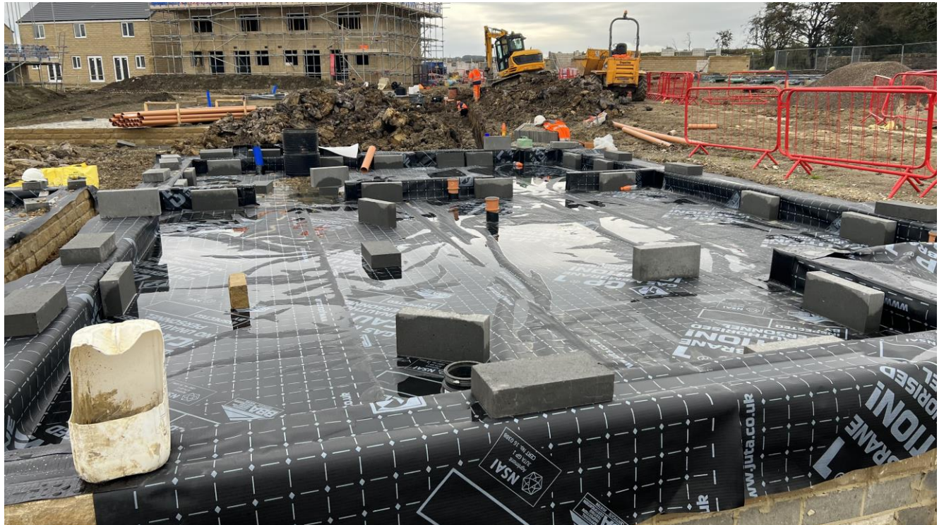
Plot 70 - Membrane layout with tophats and jointing
