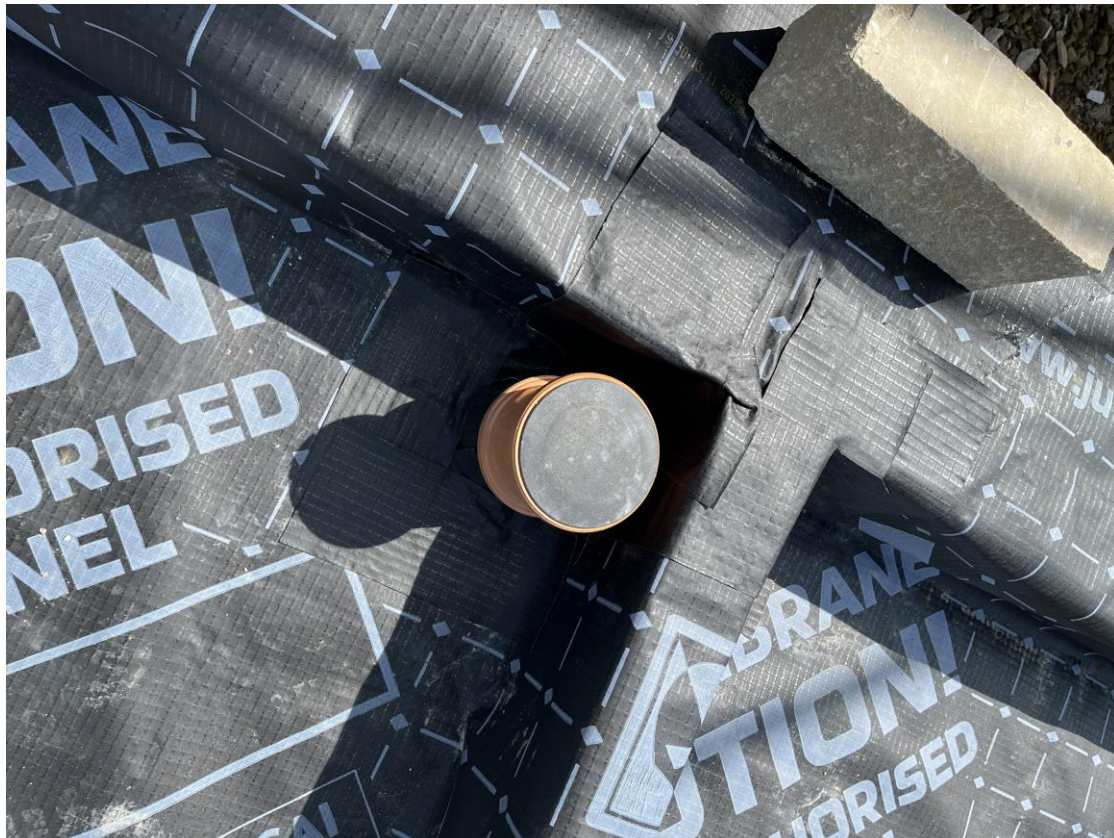
Plots 92 & 93 – Membrane layout with tophat and jointing
