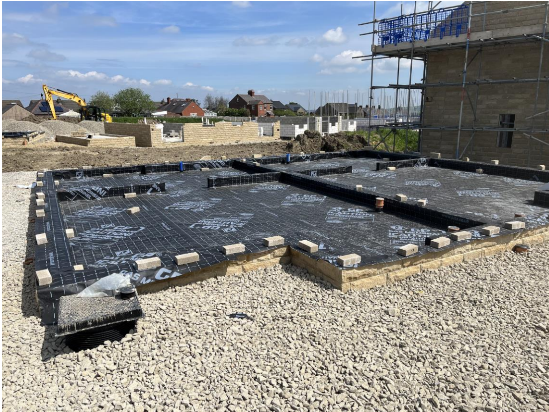
Plots 92 & 93 – Membrane layout with tophat and jointing
