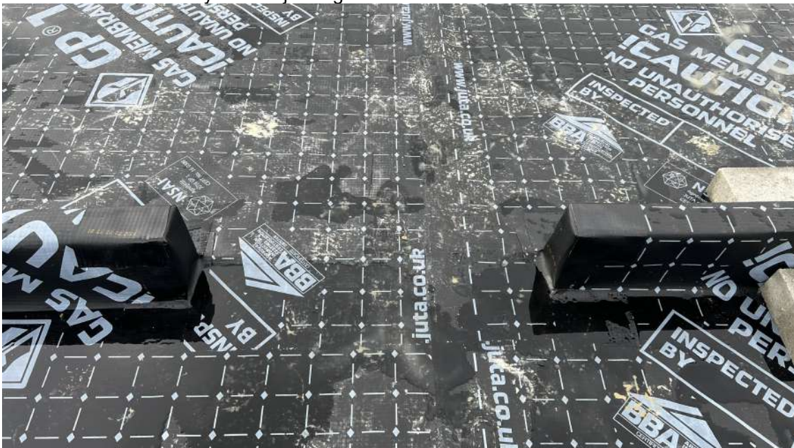
Plot 112 – Membrane layout with jointing
