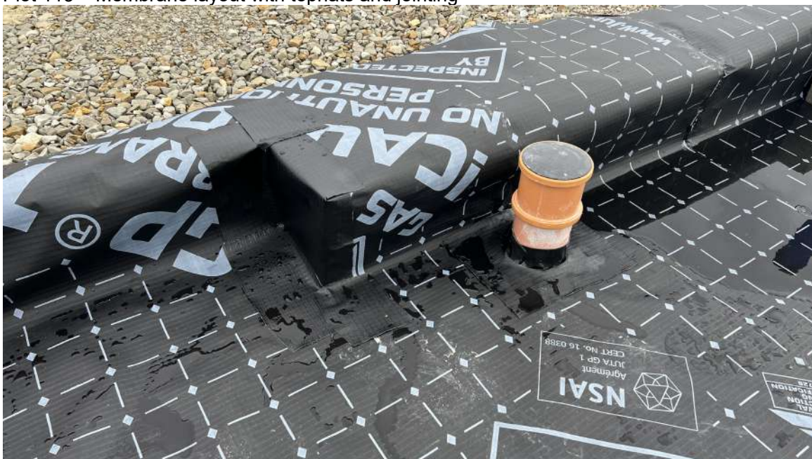
Plot 113 – Membrane layout with tophats and jointing
