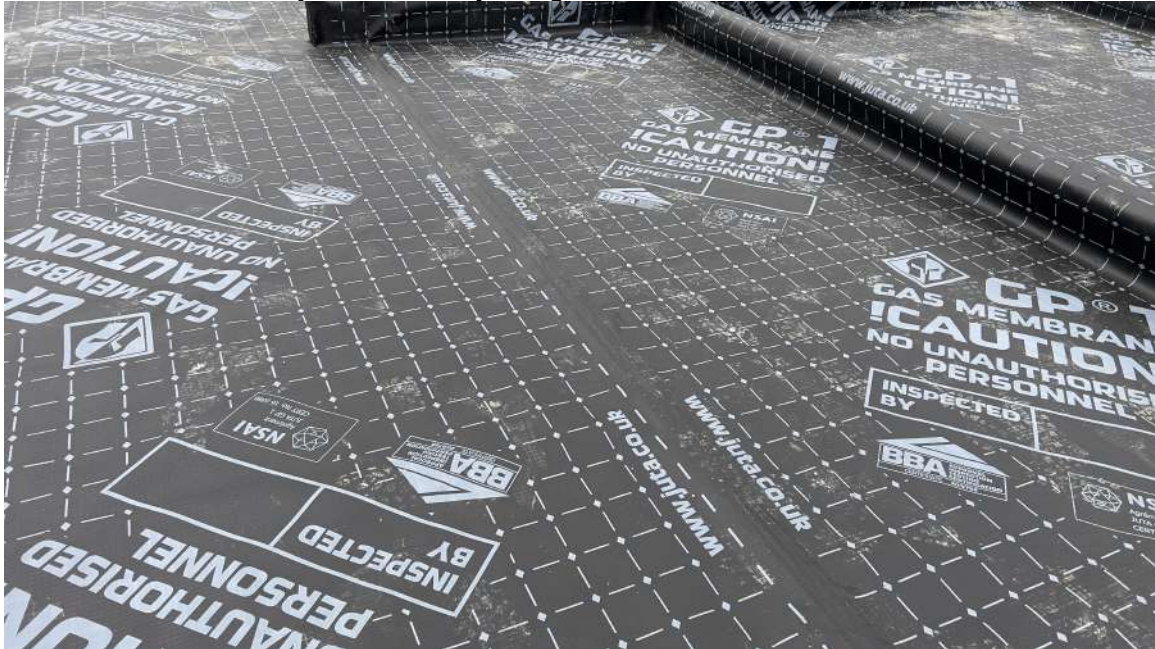
Plot 117 – Membrane layout with tophats and jointing
