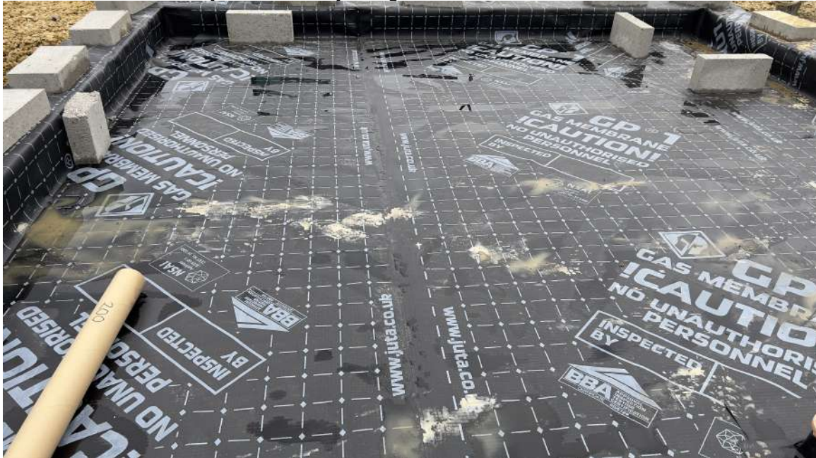
Plot 118 – Membrane layout with tophats and jointing
