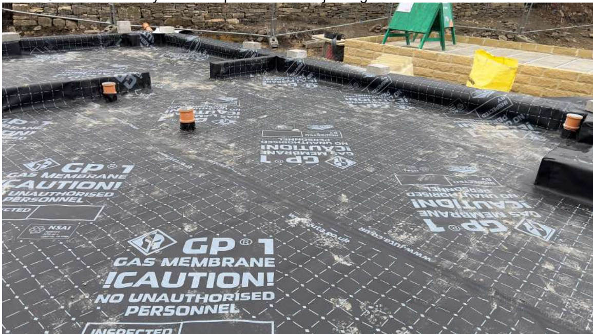
Plot 116 – Membrane layout with tophats and weld jointing
