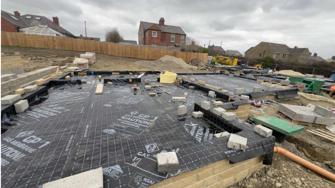
Plot 115 – Internal wall membrane layout with jointing
