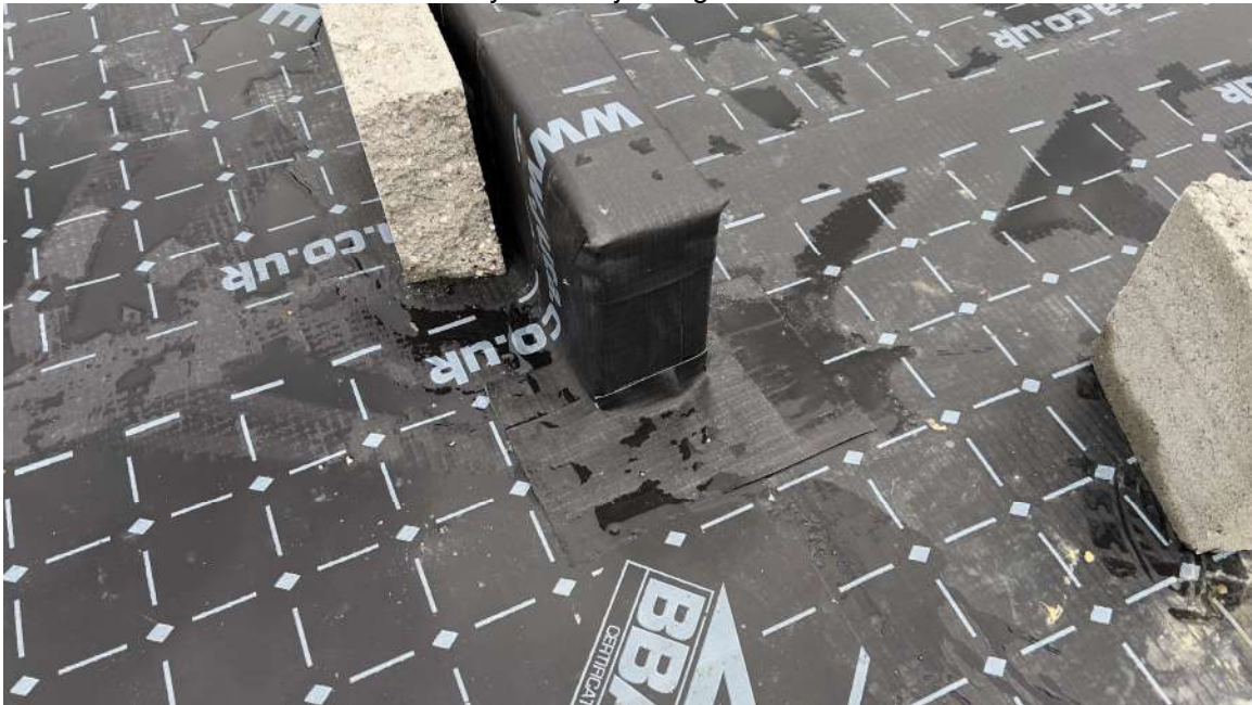
Plot 118 – Internal wall membrane layout with jointing
