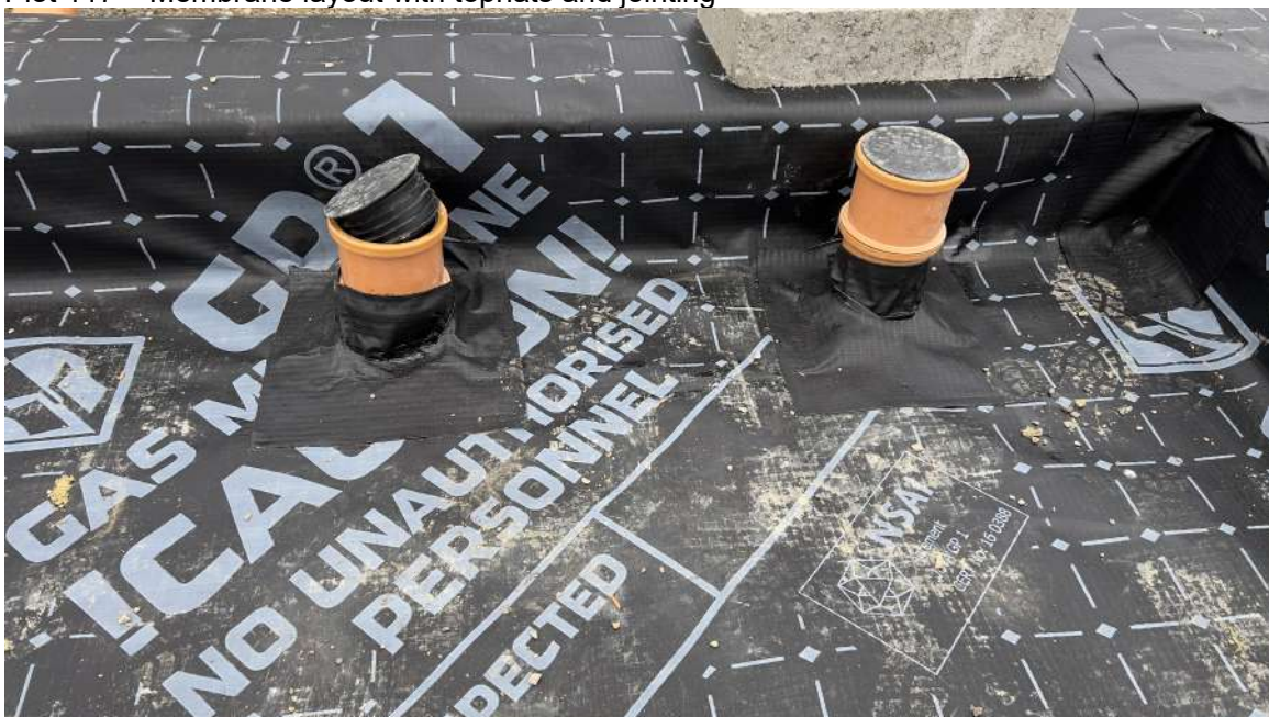
Plot 117 – Membrane layout with tophats and jointing
