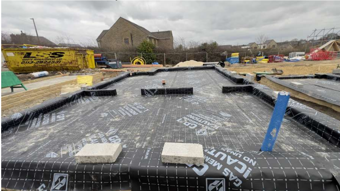
Plot 116 – Internal wall membrane layout with jointing
