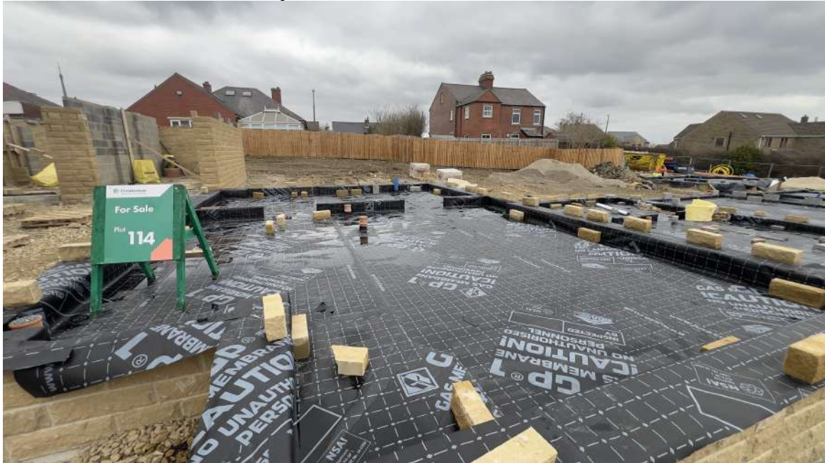
Plot 114 – Internal wall membrane layout with jointing
