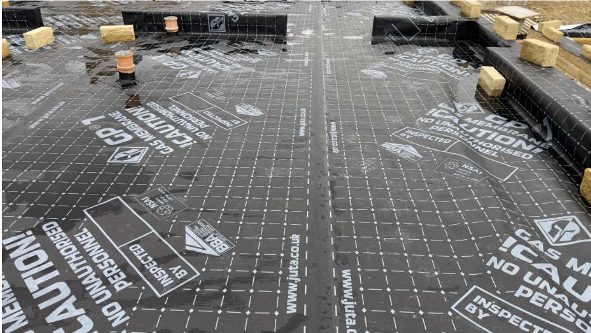
Plot 114 – Membrane layout with tophats and jointing
