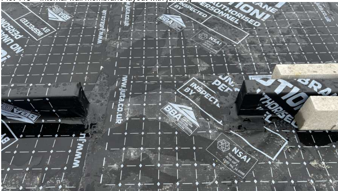
Plot 113 – Internal wall membrane layout with jointing
