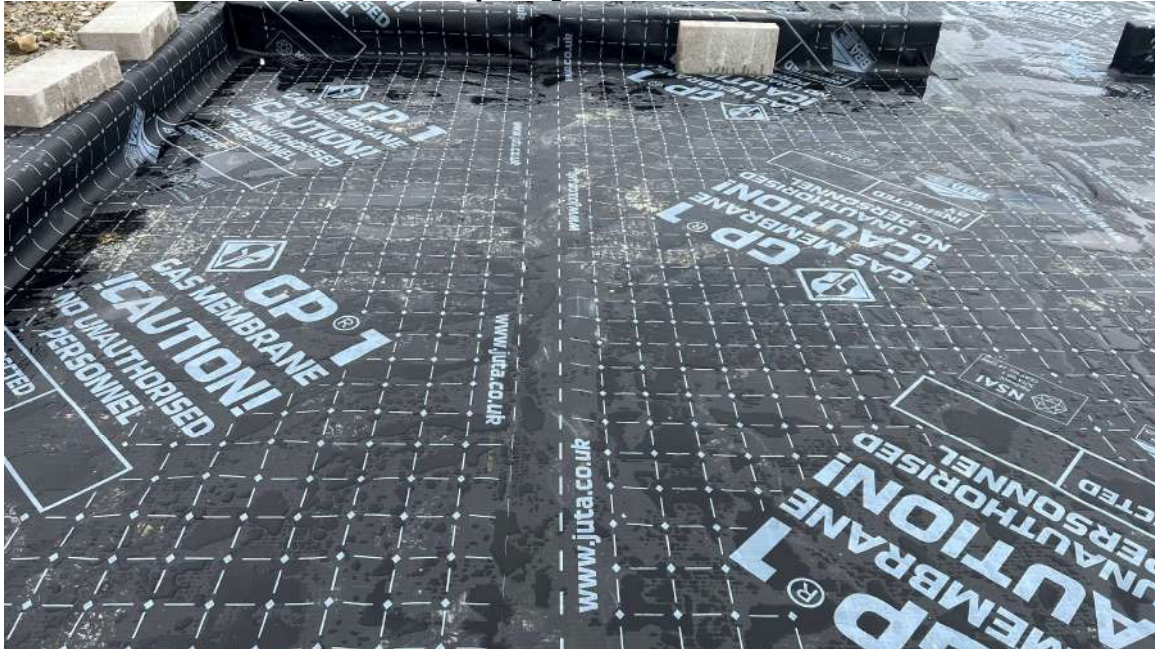
Plot 113 – Membrane layout with tophats and jointing
