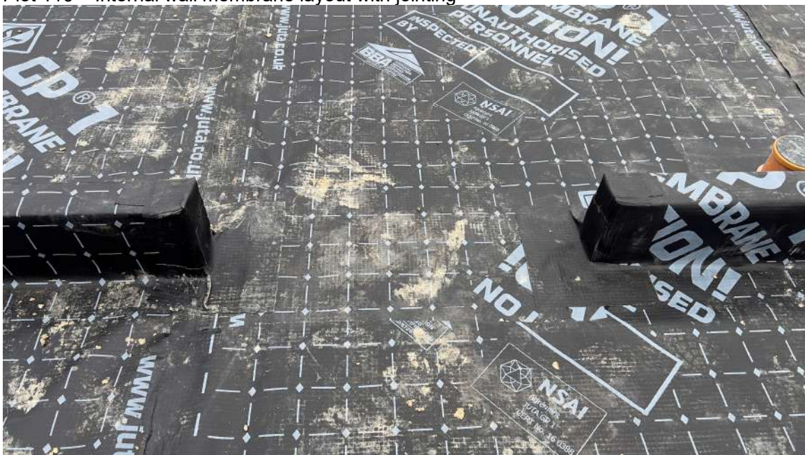
Plot 116 – Internal wall membrane layout with jointing
