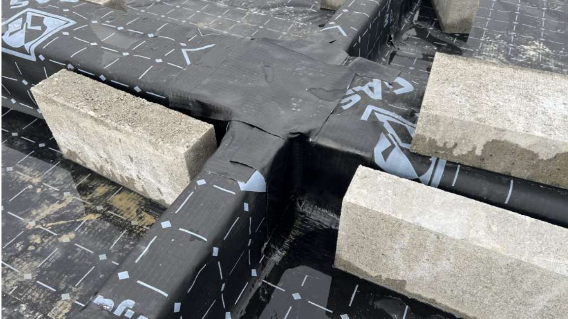
Plot 112 – Membrane layout with jointing
