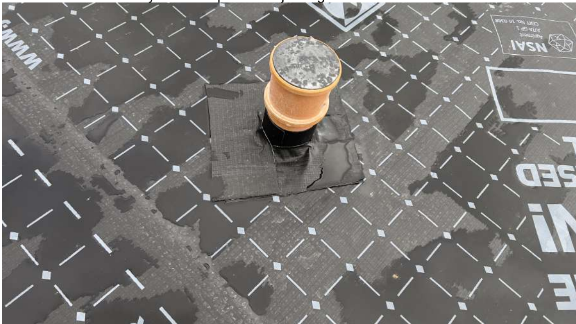
Plot 114 – Membrane layout with tophats and jointing
