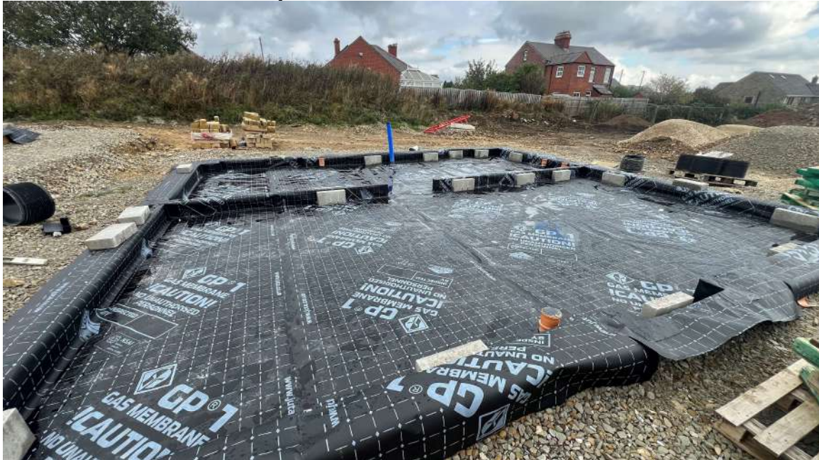
Plot 113 – Internal wall membrane layout with jointing
