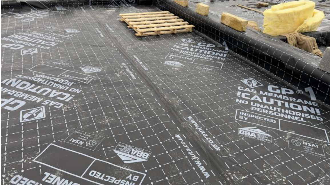
Plot 115 – Membrane layout with tophat and jointing
