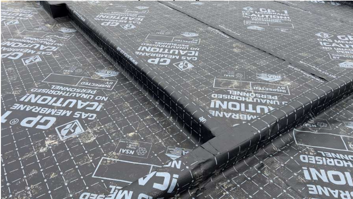
Plot 117 – Internal wall membrane layout with jointing
