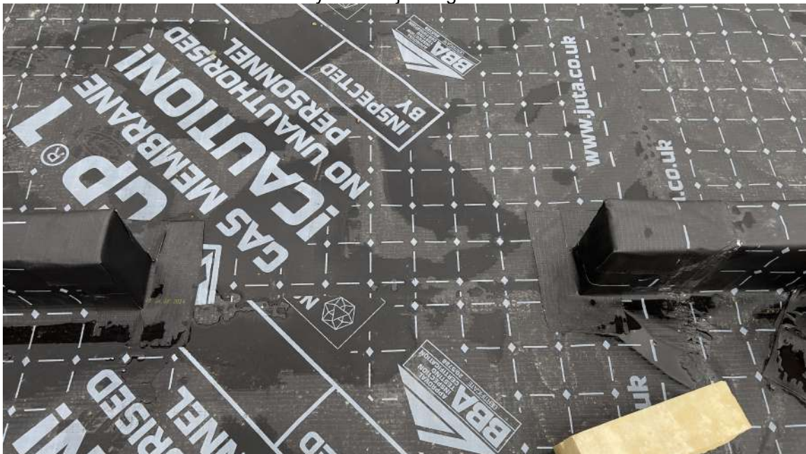
Plot 114 – Internal wall membrane layout with jointing
