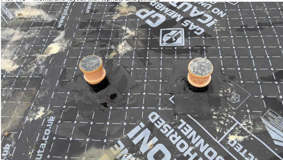
Plot 118 – Membrane layout with tophats and jointing
