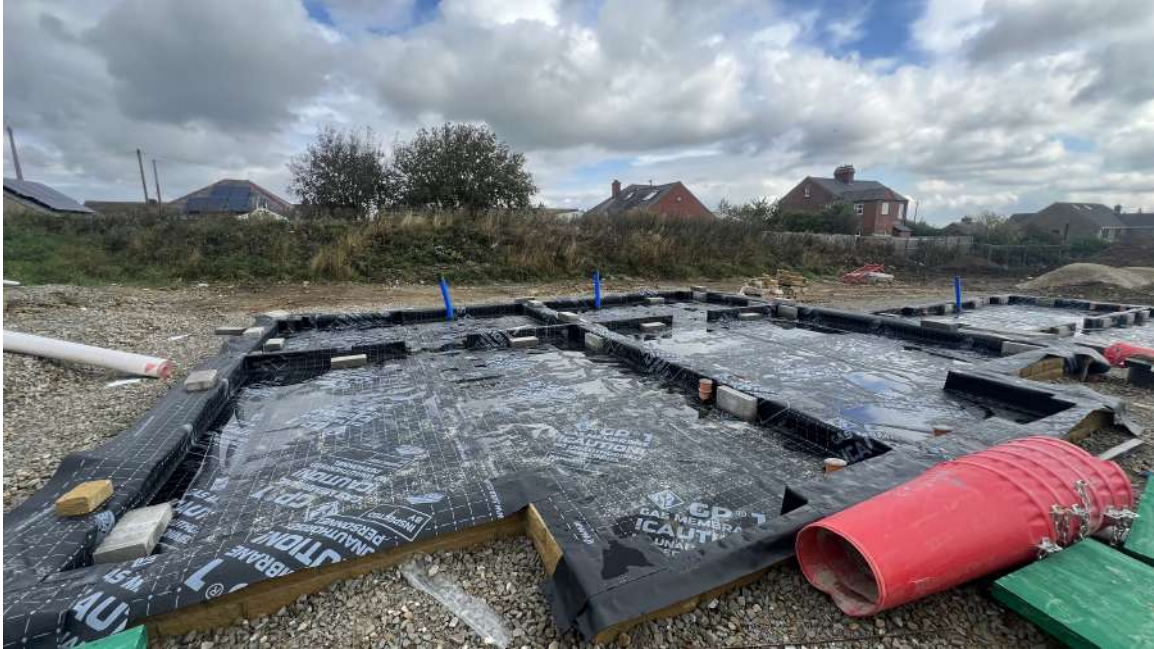
Plot 111 - Membrane layout with tophat and jointing
