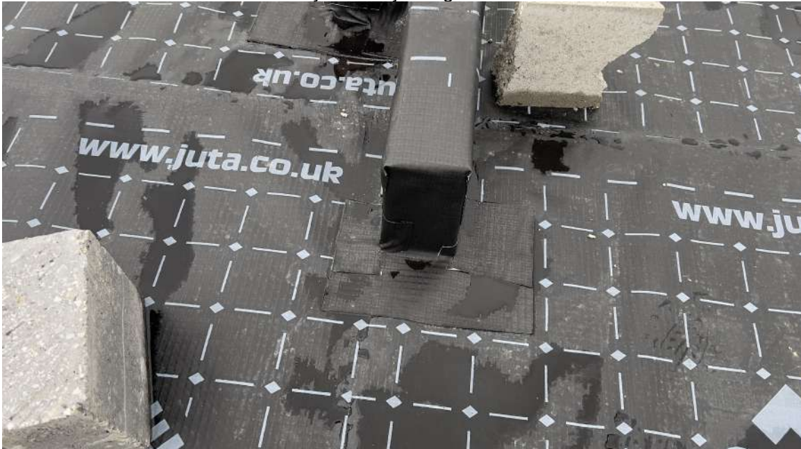
Plot 115 – Internal wall membrane layout with jointing
