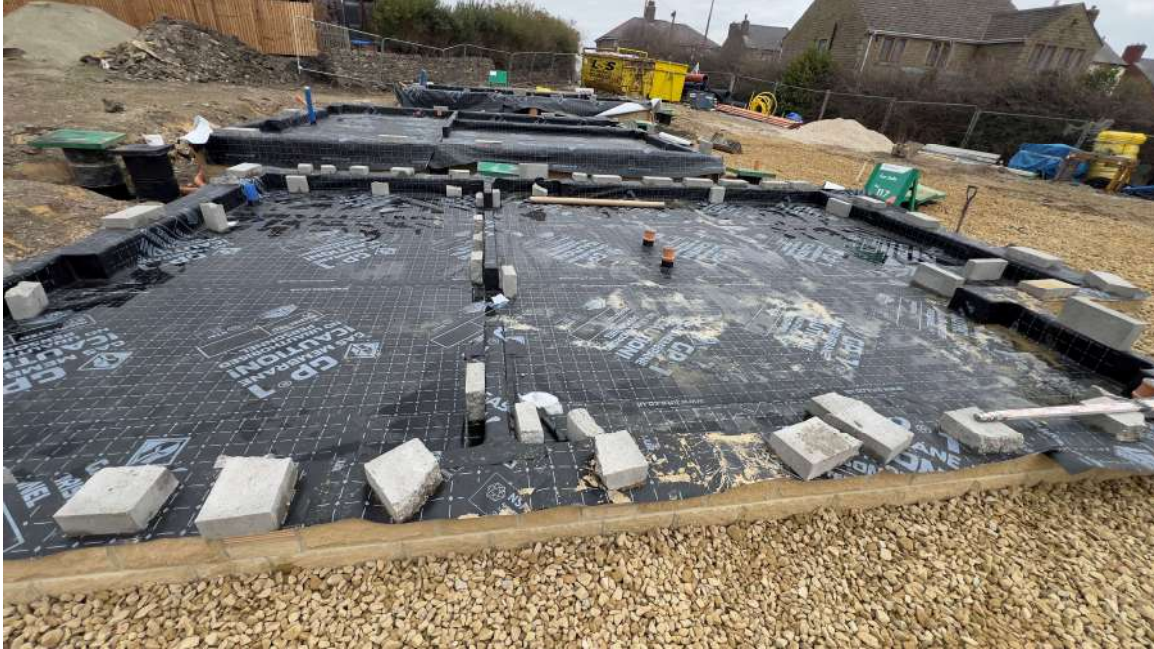
Plot 118 – Internal wall membrane layout with jointing
