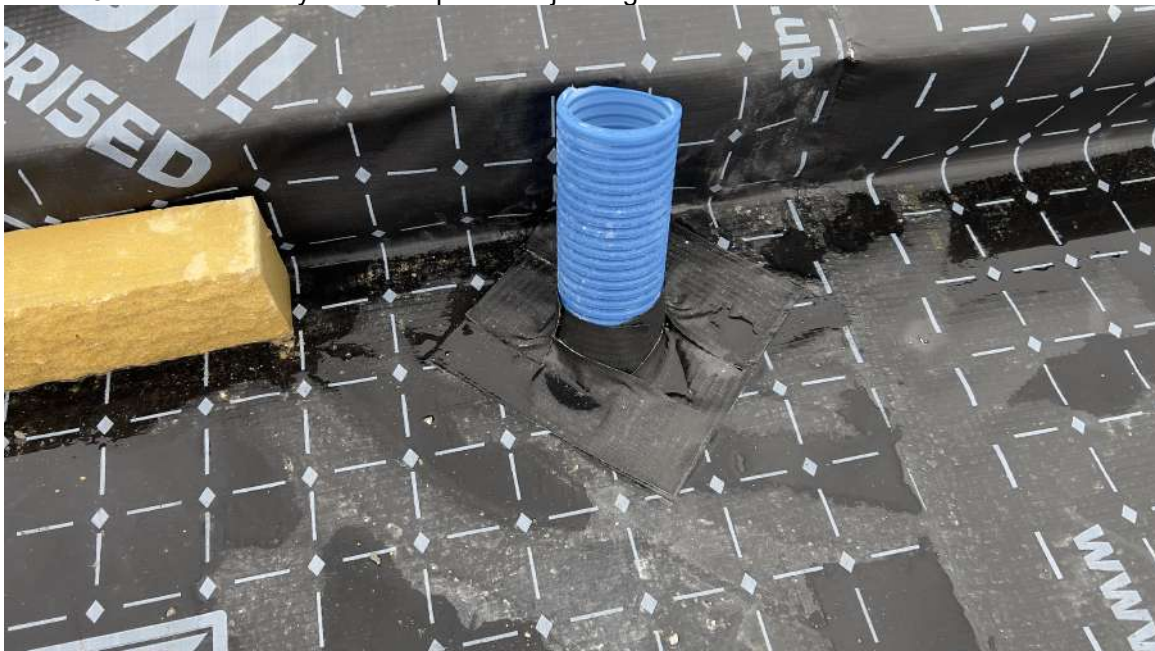
Plot 115 – Membrane layout with tophat and jointing
