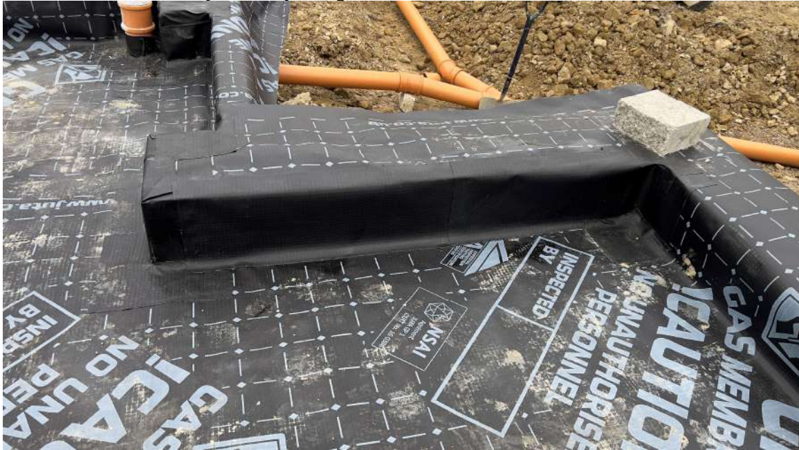
Plot 116 – Membrane layout with tophats and weld jointing
