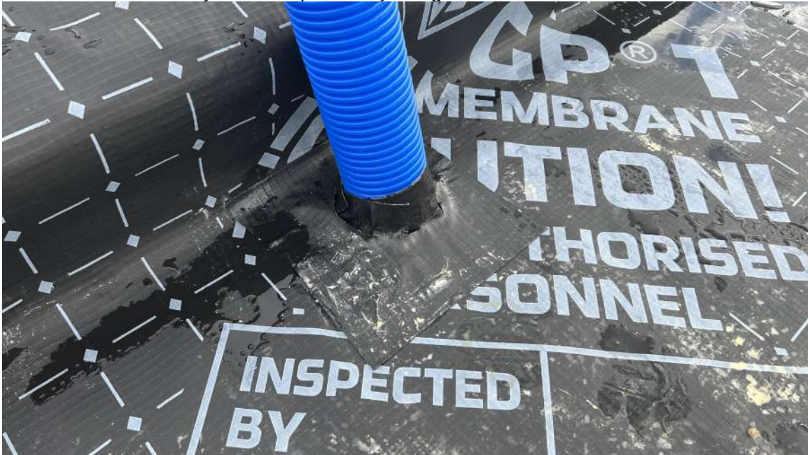
Plot 111 - Membrane layout with tophat and jointing
