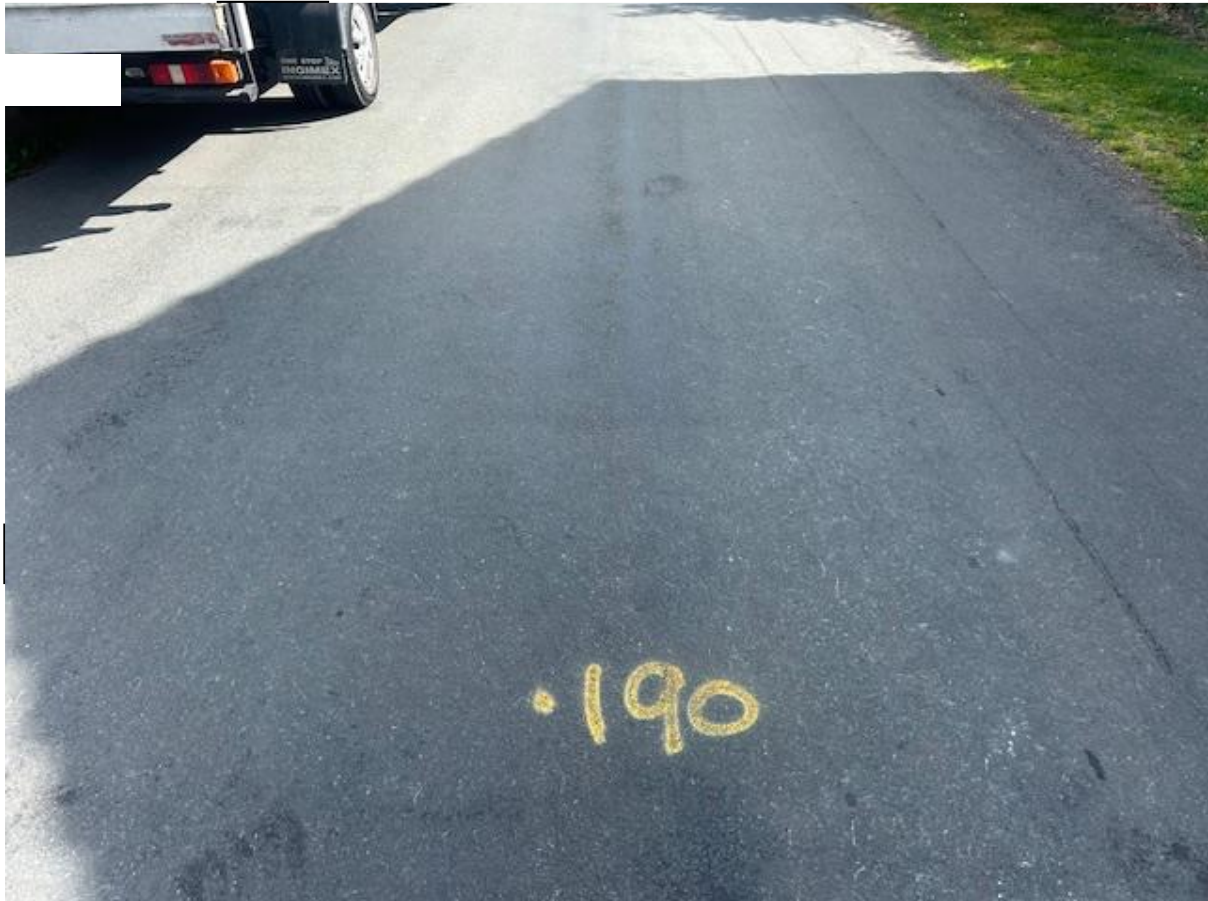
Comments – trench reinstatement along southern flank of Denby Lane.
