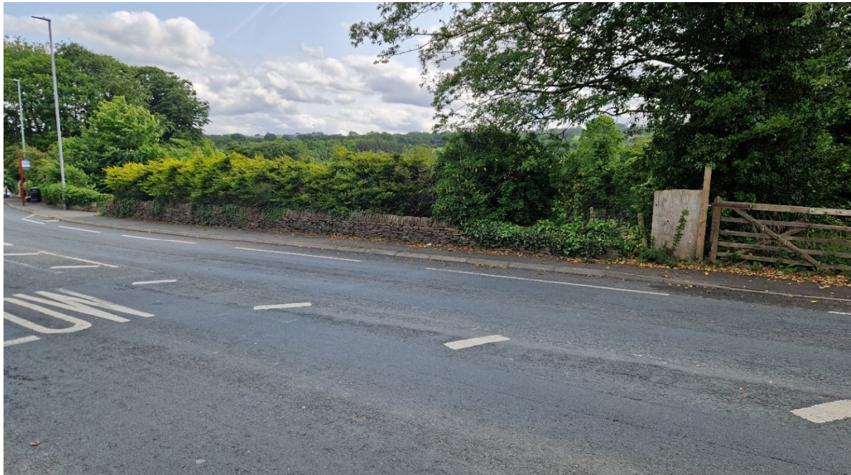
Figure 1. View of the wall
