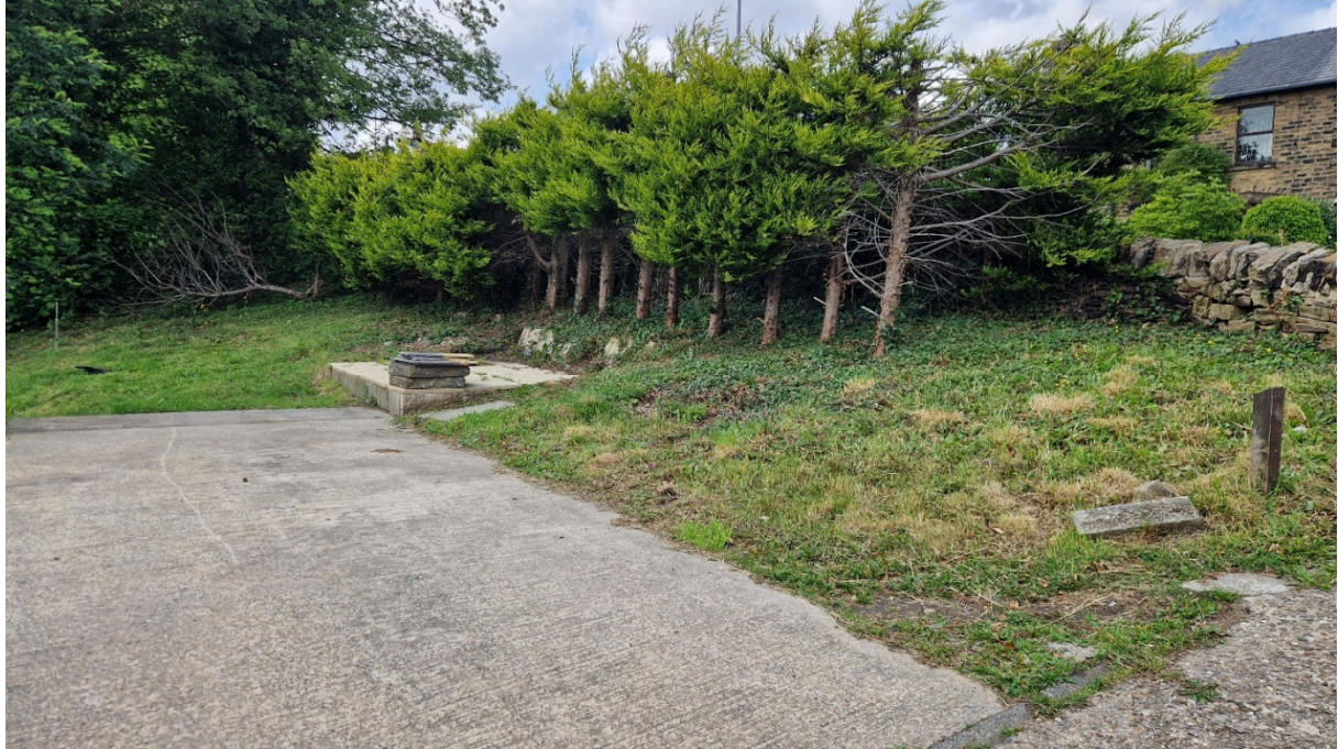
Figure 2. View of the rear of the wall
