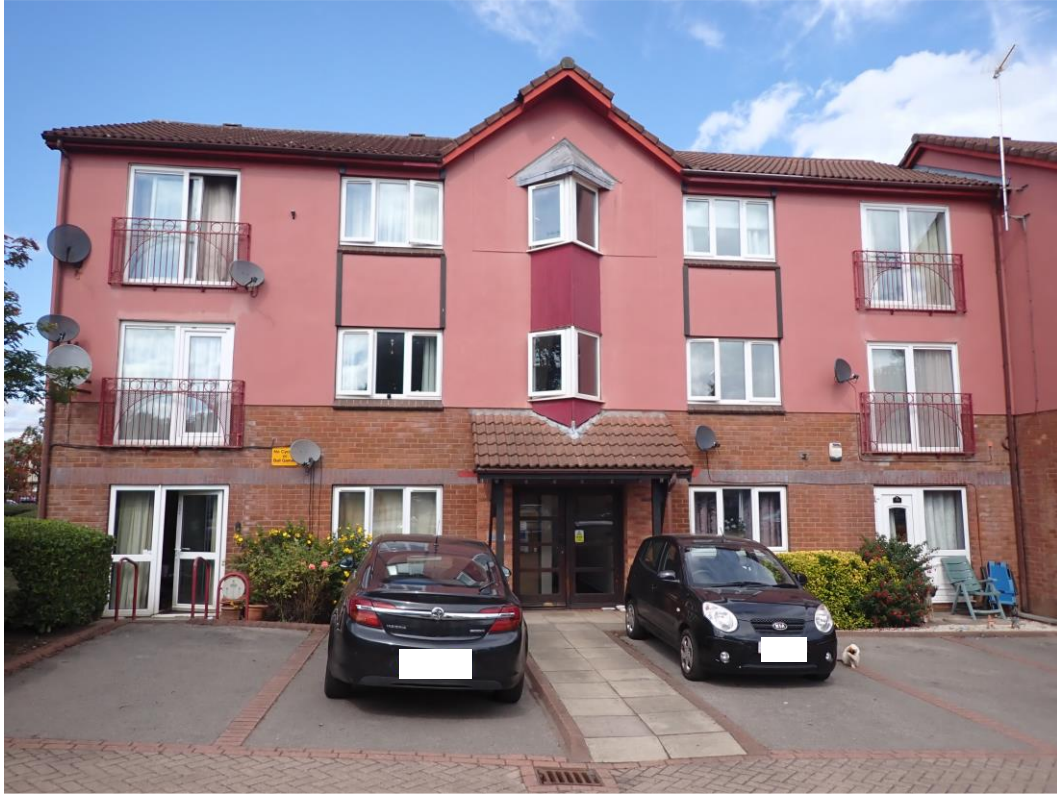
Photograph 2—Typical Common Entrance Doors and Painted Timber Bay
