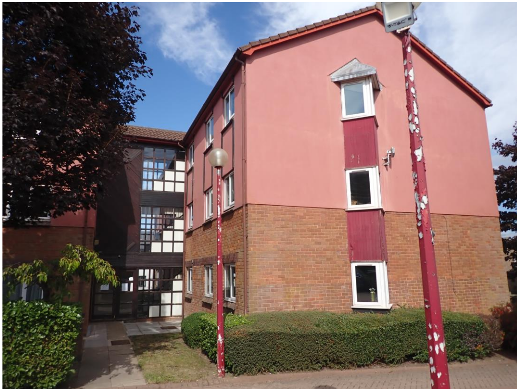
Photograph 1—Typical Curtain Walling and Painted Timber Bay
