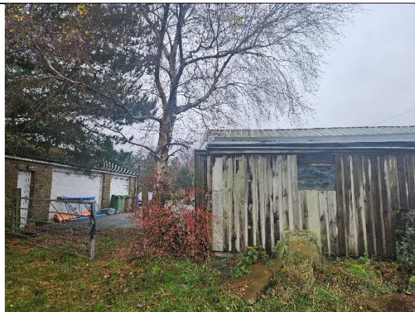
Photo 2: Location of B2 and brash piles adjacent.
