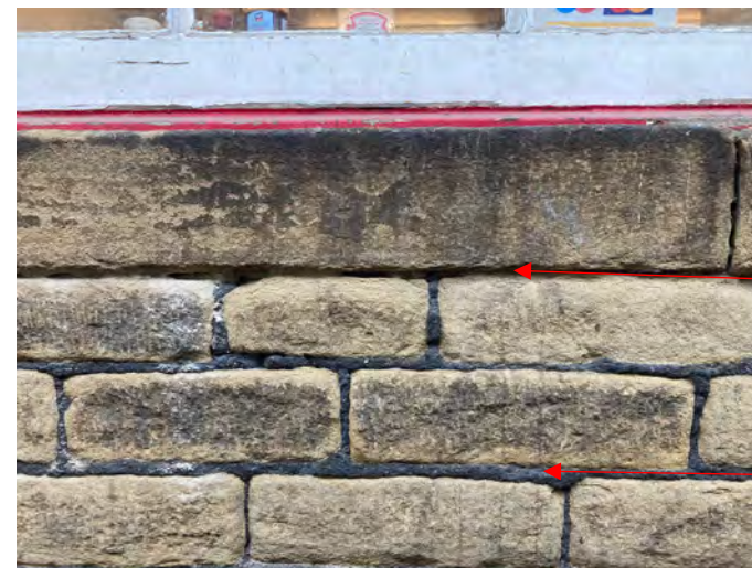
Sample 2: Underlying early mortar
