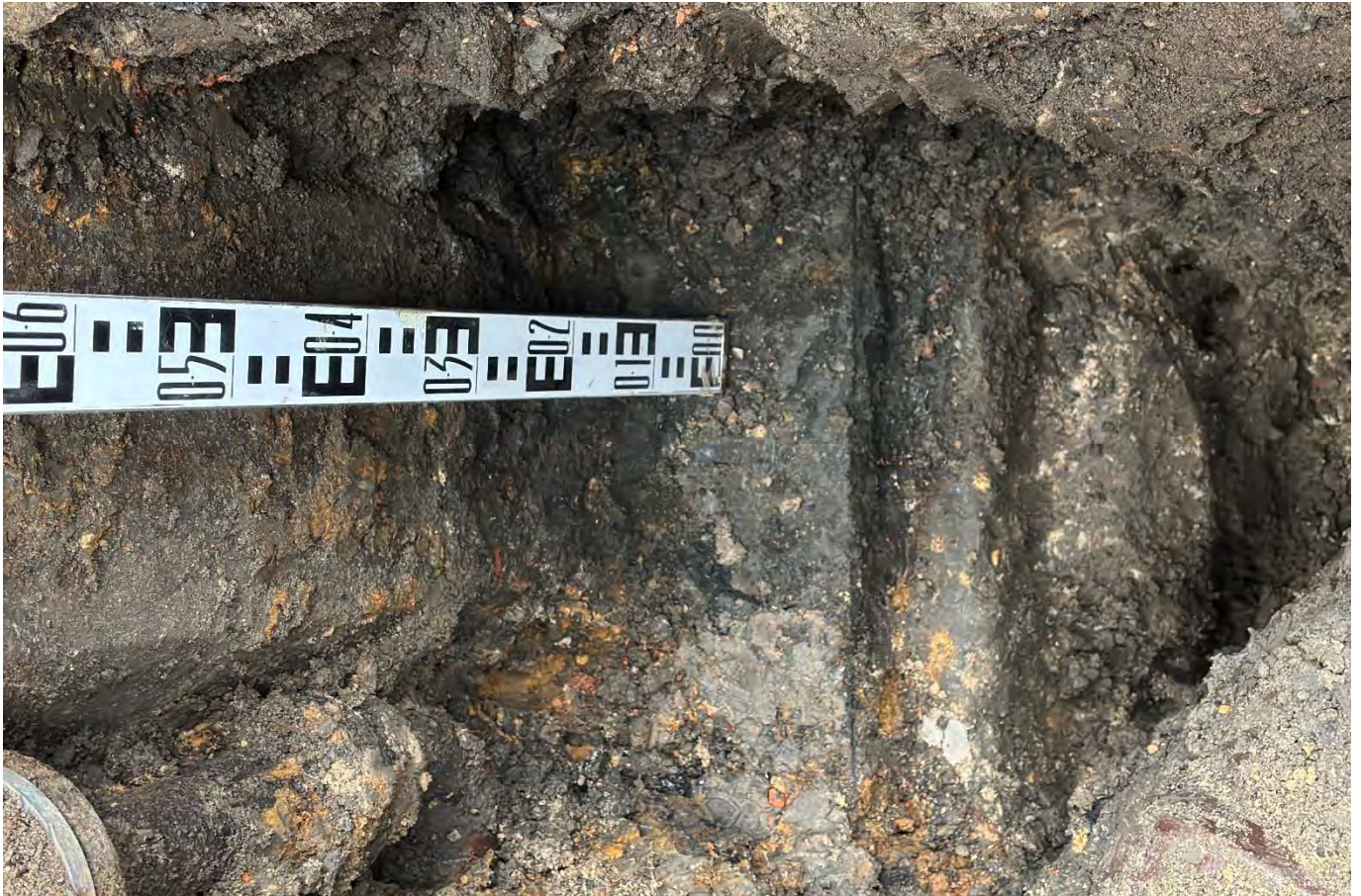
TP15: Staff resting of steel pad set at the base of supporting column. Pad founded on sandstone boulders. Note ceramic drain to the bottom right
