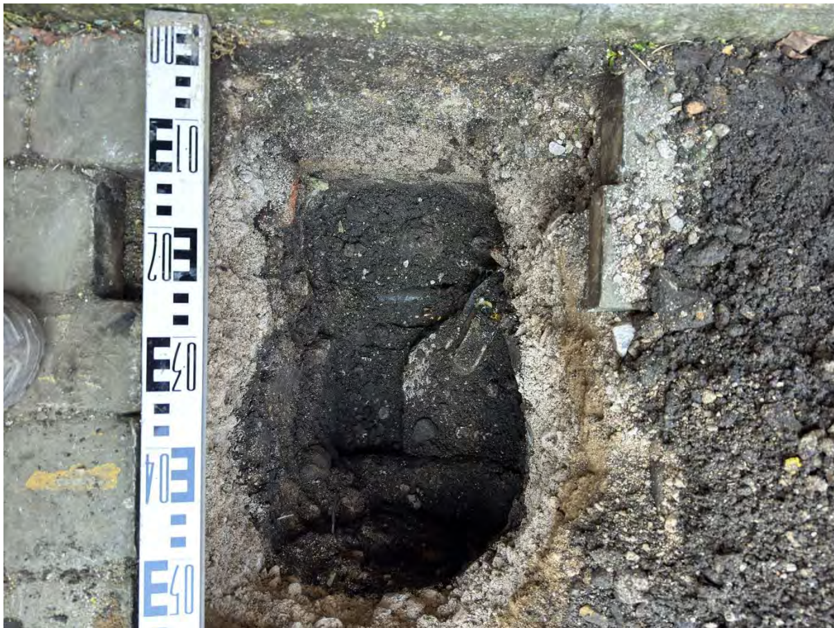
TP02-c: Showing buried electrical services repair at 0.77mbgl
