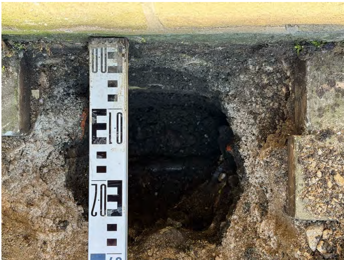
TP02-b: Showing buried electrical services extending along building alignment
