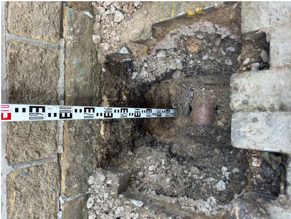
TP02-a: Showing buried ceramic drains extending along building alignment
