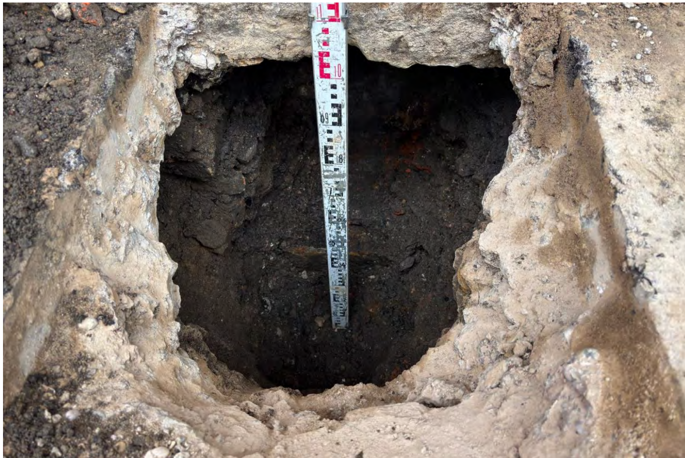
TP07: Showing base plate constructed at the base of support column
