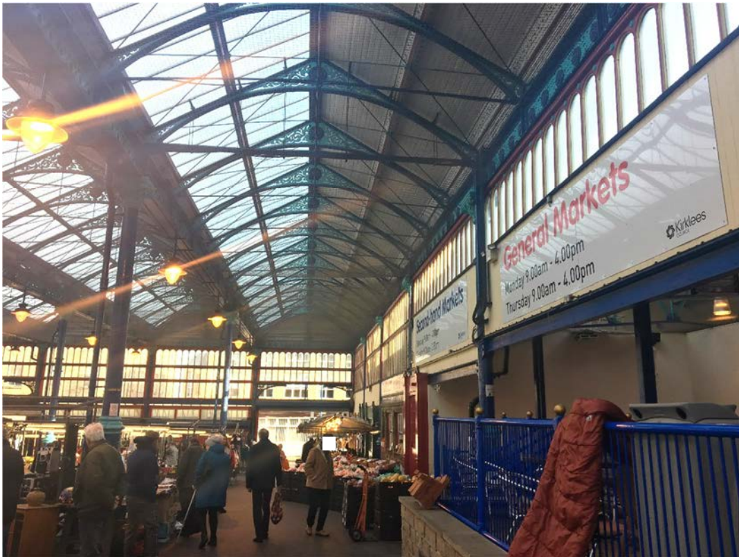
Figure 14. View of the interior of the Wholesale Market looking east, with the wall of the building adjoining the market's south wall on the right of photograph.
