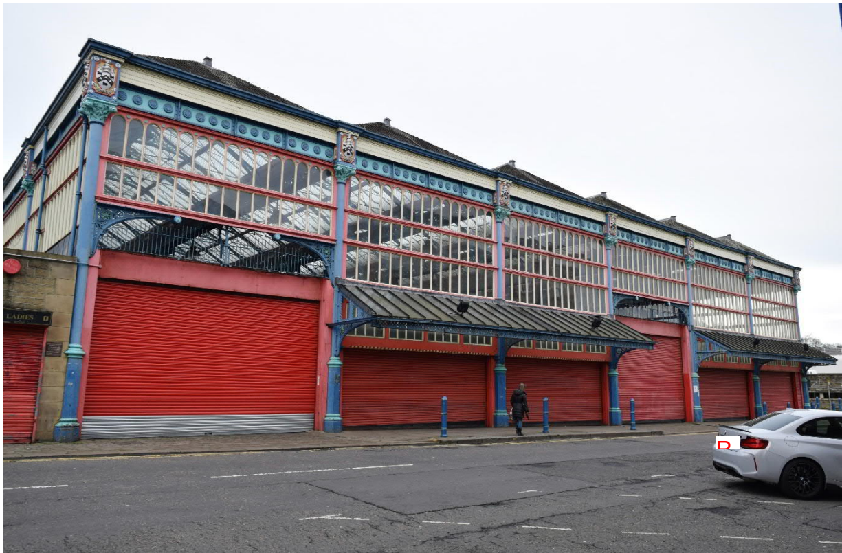
Figure 7. The east elevation of the Wholesale Market, looking north-west.
