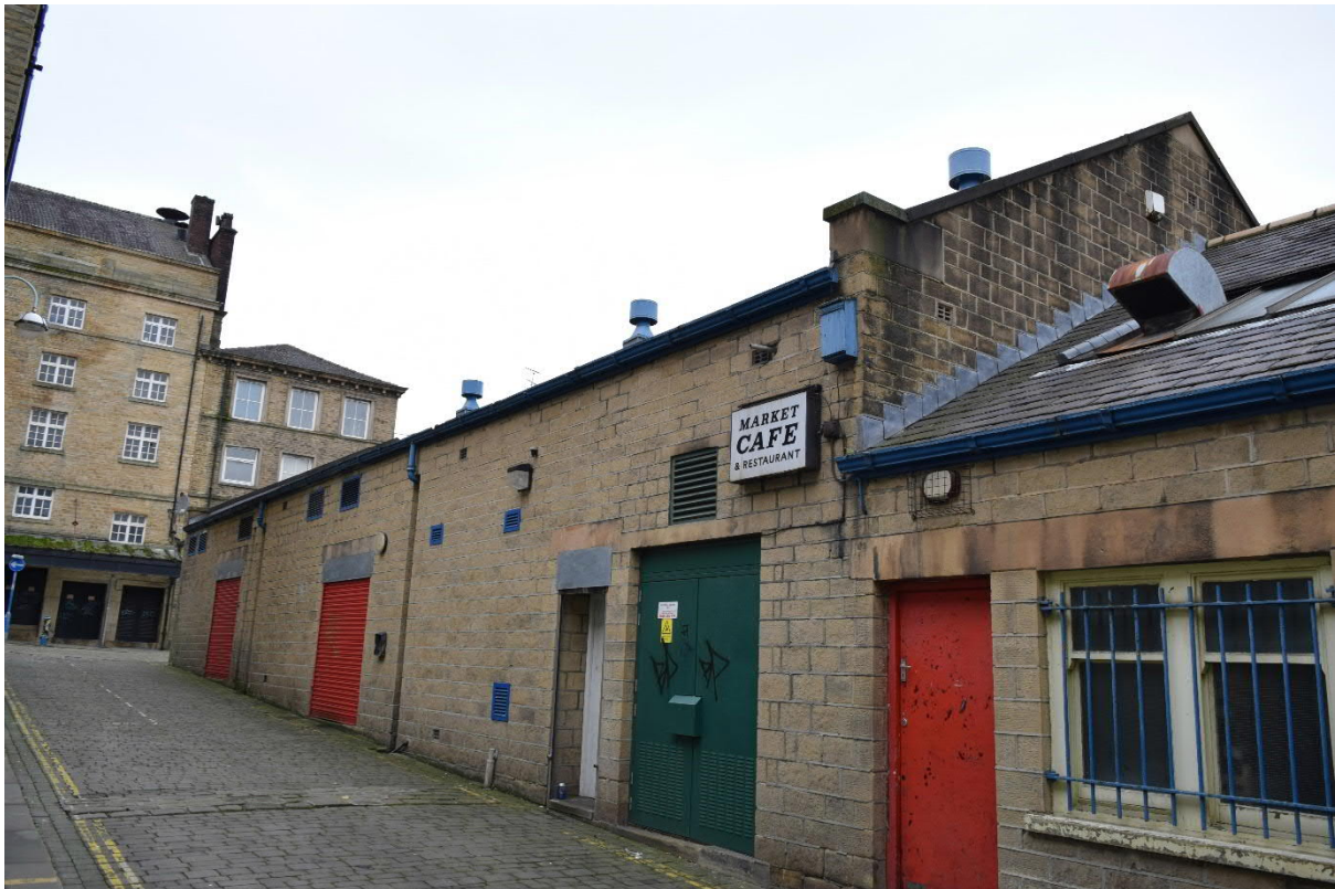
Figure 19. West end of the south elevation of the 1930s building erected on the south side of the market.
