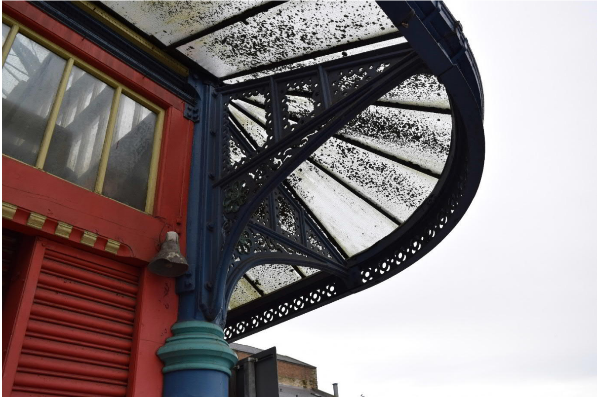
Figure 11. Detail of the curved verandah on the Wholesale Market's north-east corner.
