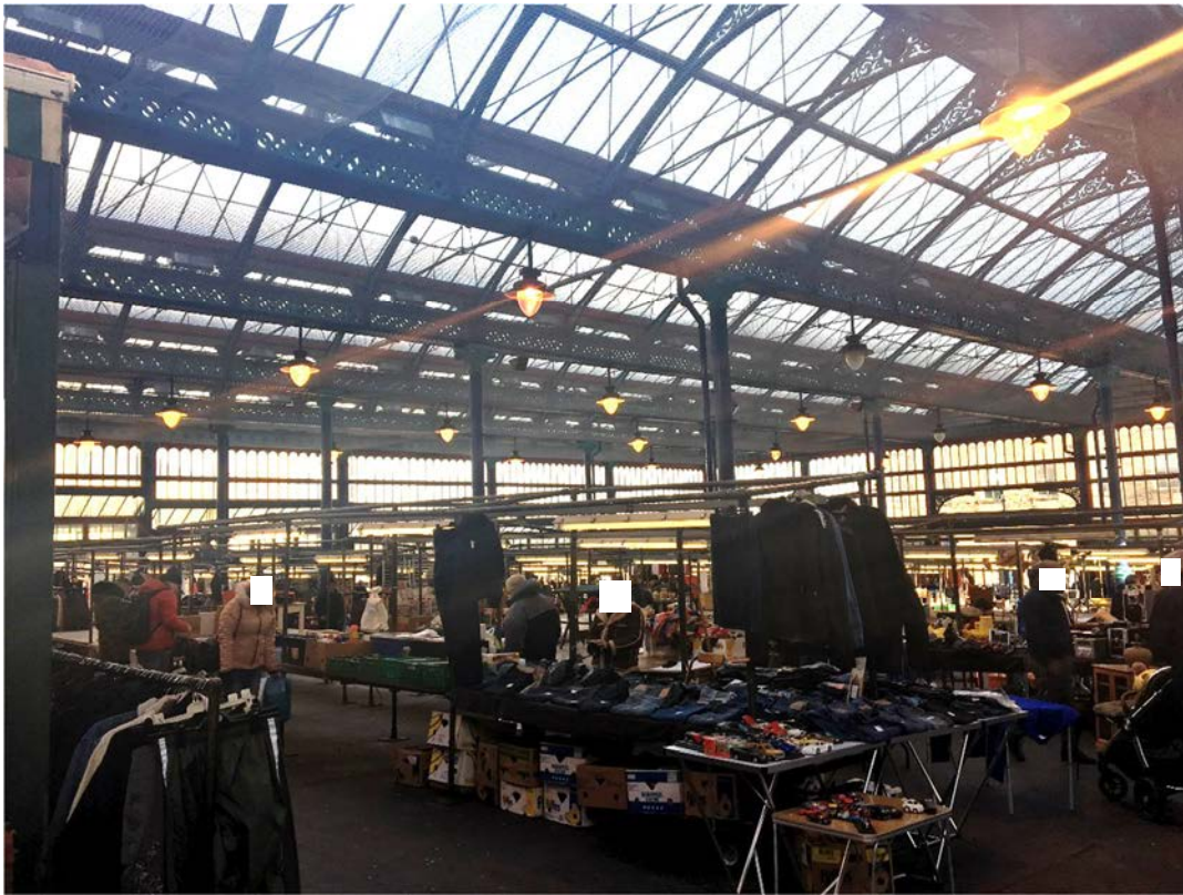
Figure 13. View of the interior of the Wholesale Market showing the north light roof glazing.
