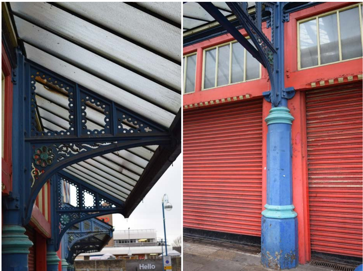
Figure 12. Detail on the ironwork on the external elevations of the Wholesale Market.
