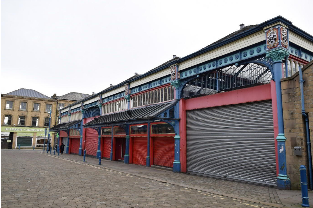
Figure 9. West elevation of the Wholesale Market, looking north-east.
