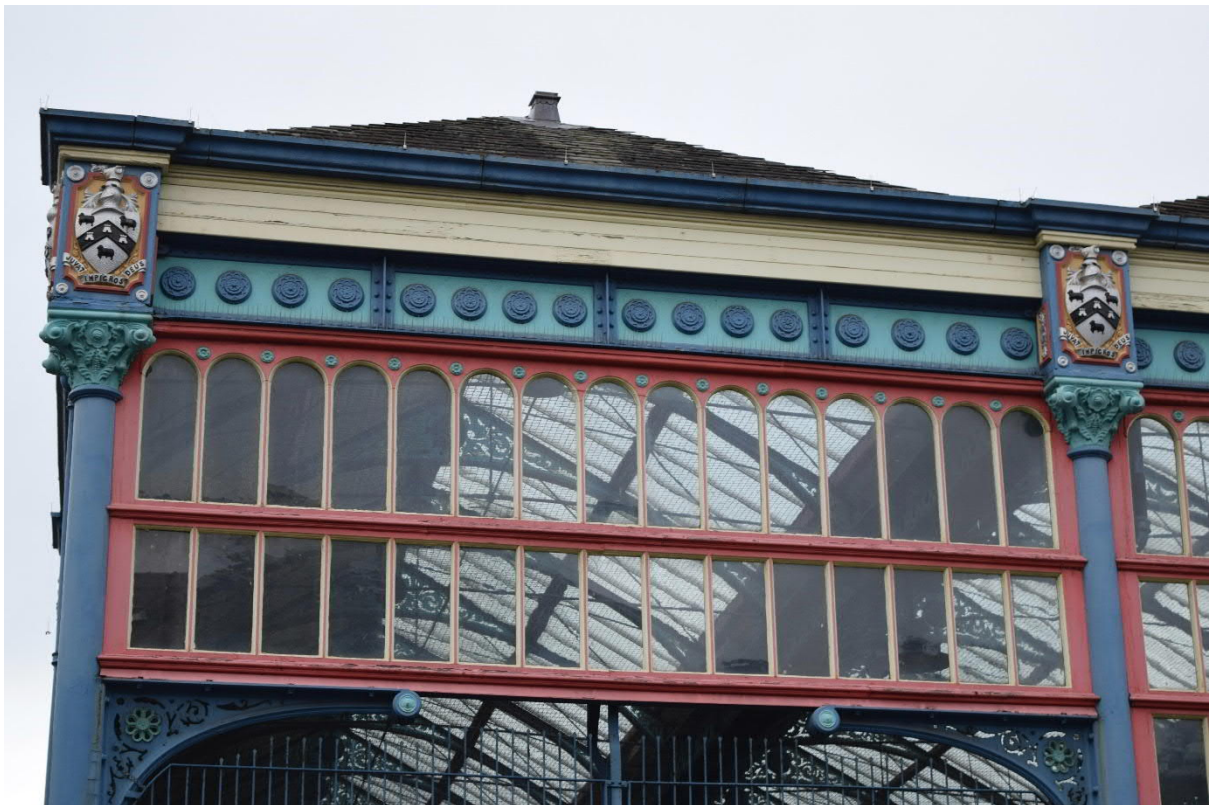
Figure 10. Detail of the ironwork on the external elevations of the Wholesale Market.
