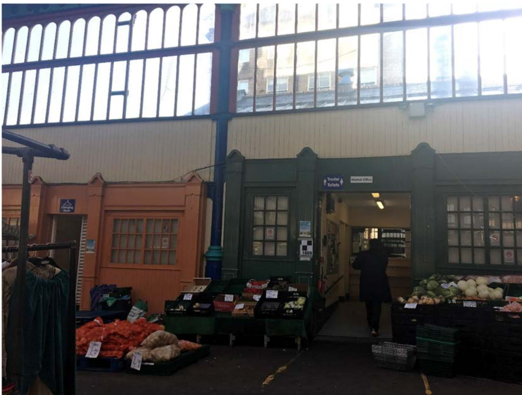
Figure 16. View of applied faux shop frontages on the south wall of the market hall leading to the building adjoining its south side.
