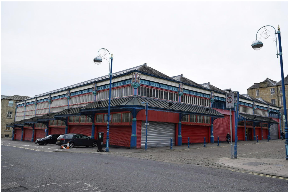
Figure 3. View south-east along Brook Street showing the Wholesale Market, the historic style of street lighting and the use of setts to the parking bays on the market's north side.
