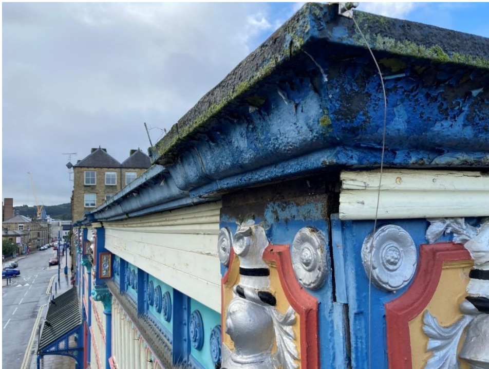
16. Section of trim removed during inspection
