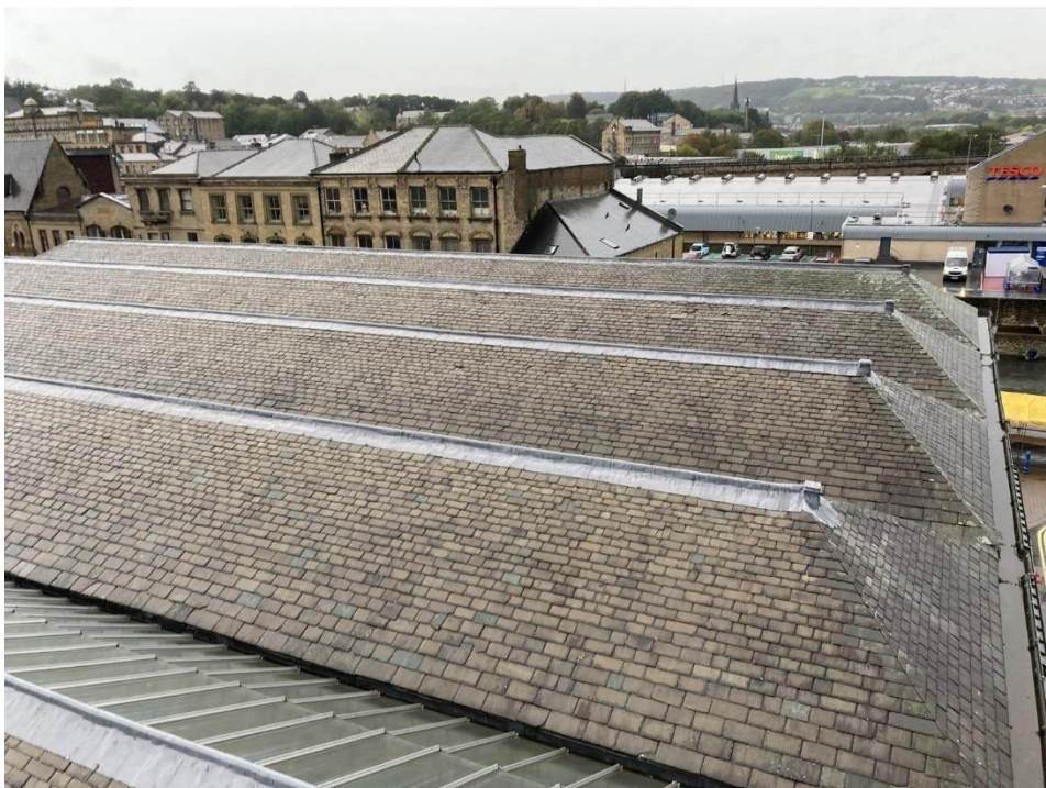
4. General view of slated pitches of roofs –as above
