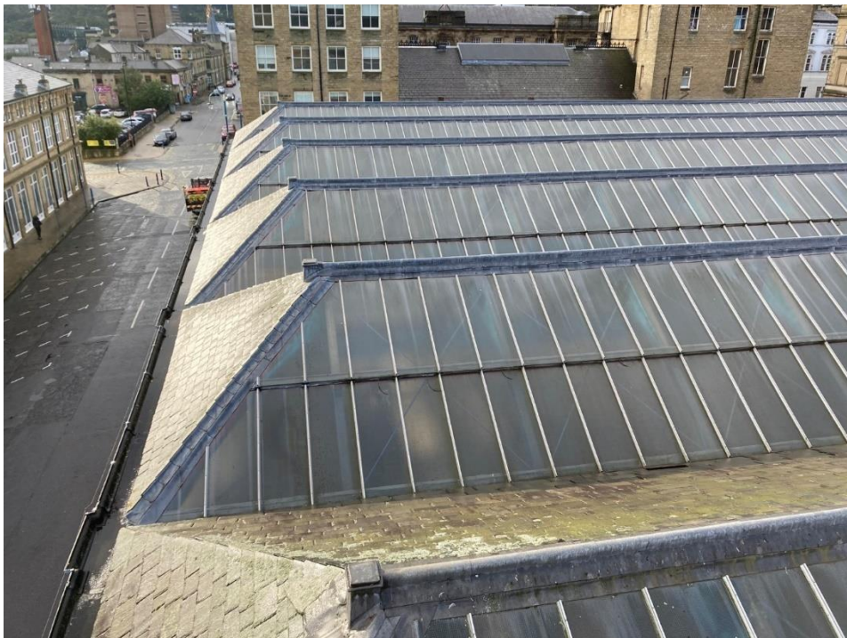
12. General view of glazed pitches of the roof
