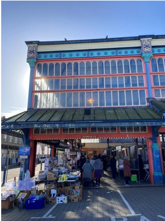
34. Bay 6 of Byram Street – a more exposed location with a corresponding higher amount of repairs
