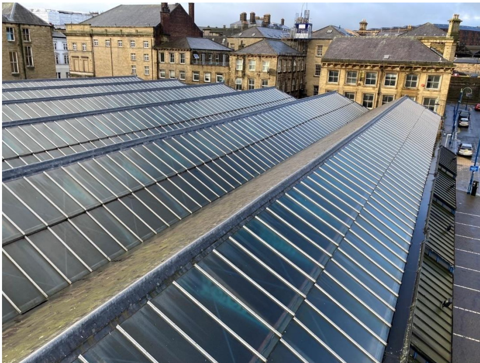
14. General view of glazed pitches of the roof
