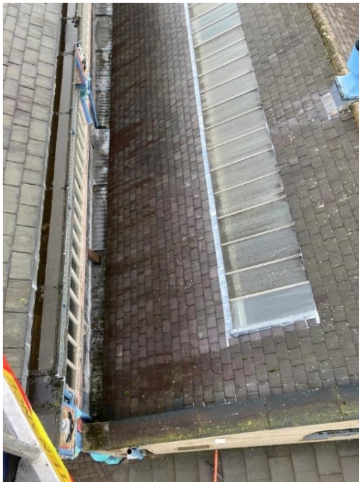
23. General view of upper end of stone extension and Back Street elevation of Market
