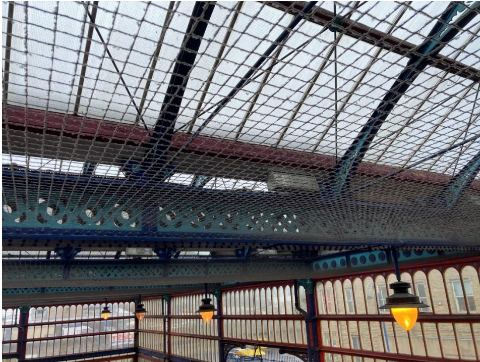
30. Closeup of netting showing general build up of soil
