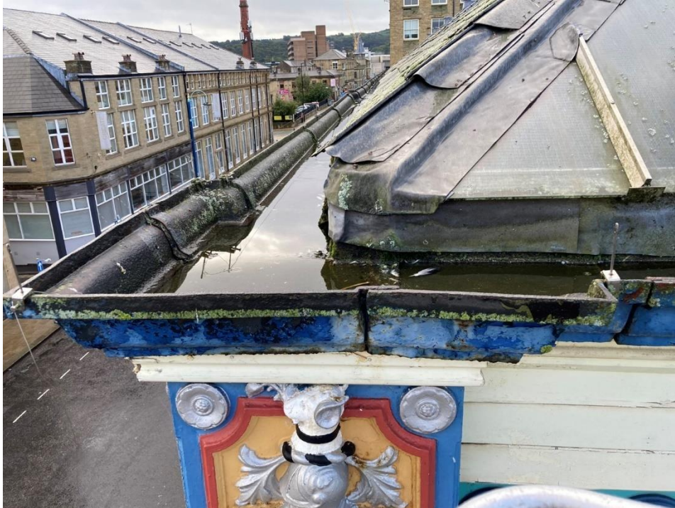
15. Typical condition of perimeter gutters
