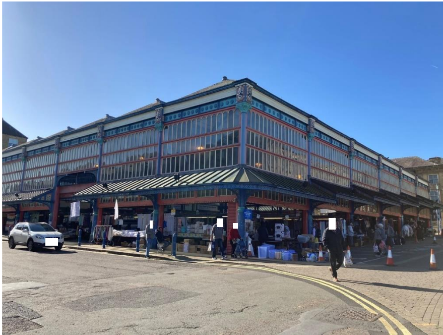
1. General view of Huddersfield Open Market from the corner of Lord Street and Brook Street
