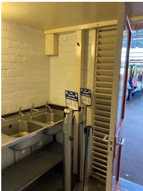
37. Typical condition of changing rooms
