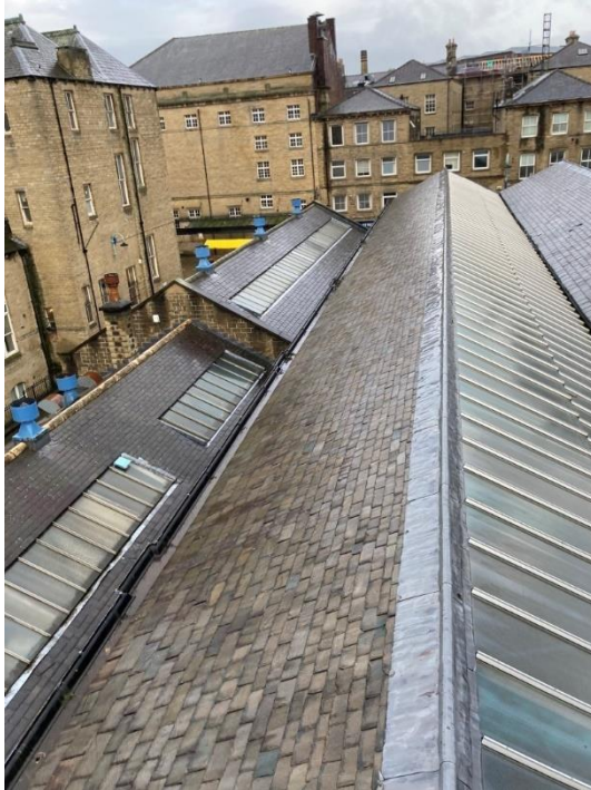
5. General view of stone extension roofs (ER1 and ER2)
