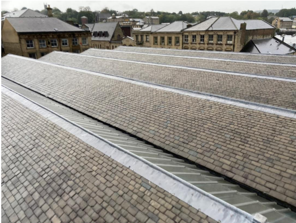
3. General view of slated pitches of roofs – generally in good condition, with a handful of slipped and missing slates
