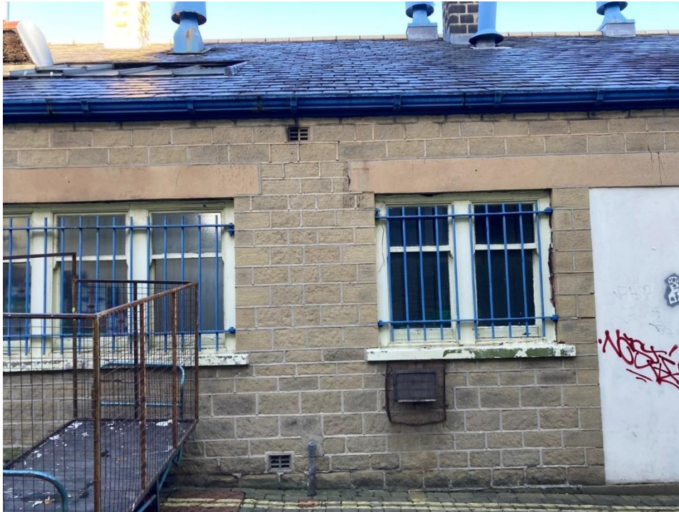
26. Back Street elevation of stone extension – typical condition of windows
