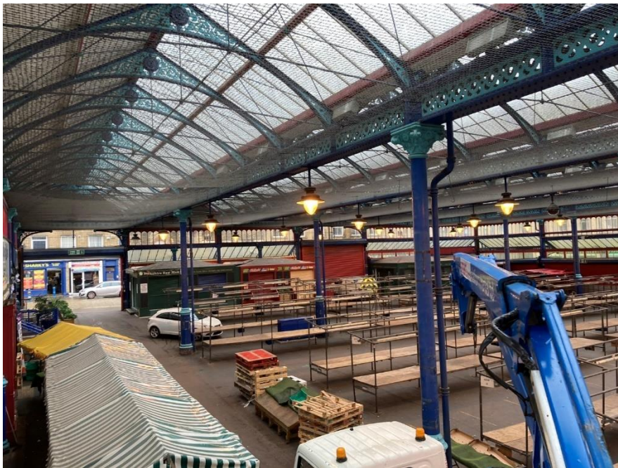
2. General internal view
