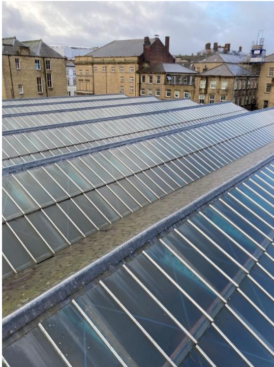
13. General view of glazed pitches of the roof
