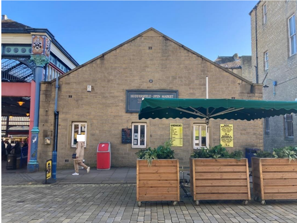
24. Byram Street elevation of stone extension
