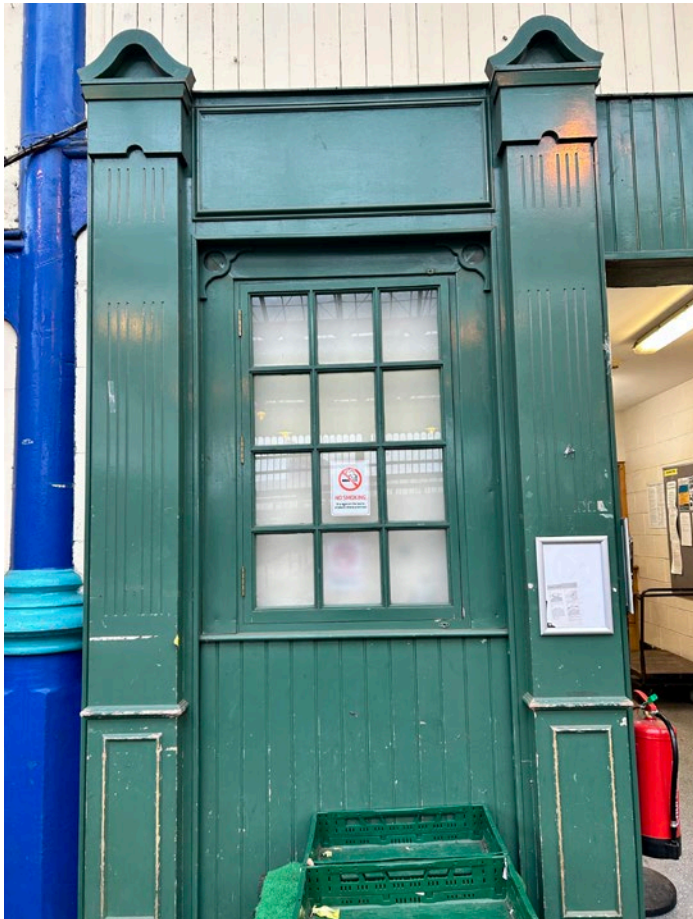
Photograph inside the existing market hall
