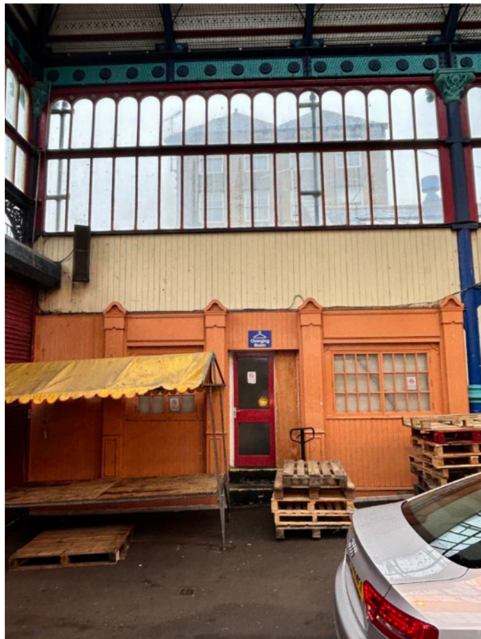
Photograph inside the existing market hall
