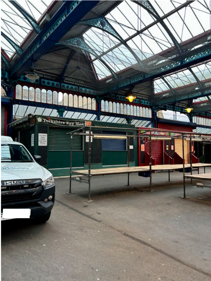
Photograph inside the existing market hall
