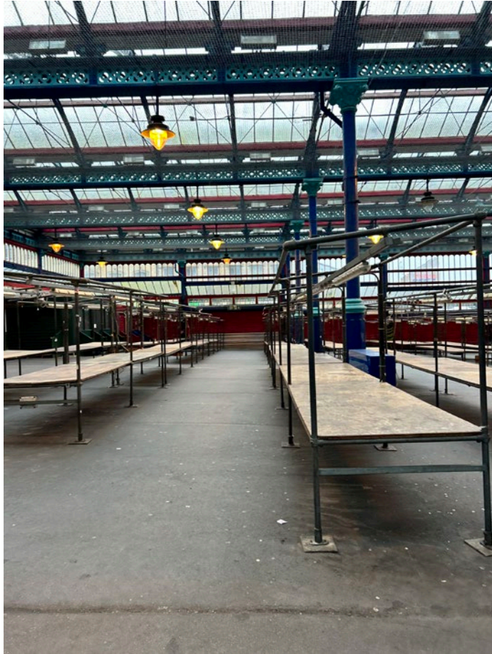
Photograph inside the existing market hall
