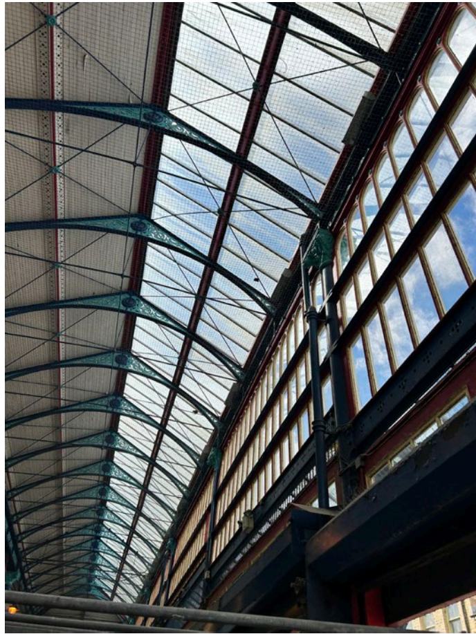
Photograph inside the existing market hall
