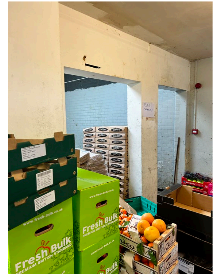
Photograph inside the existing market annexe
