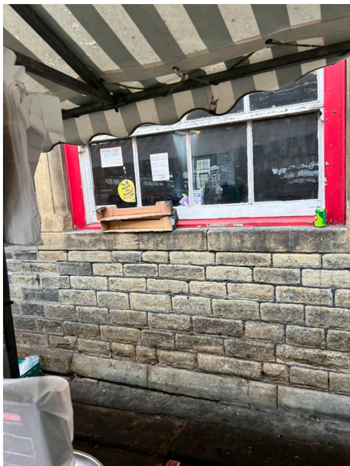
Photograph inside the existing market hall
