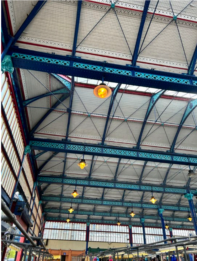
Photograph inside the existing market hall
