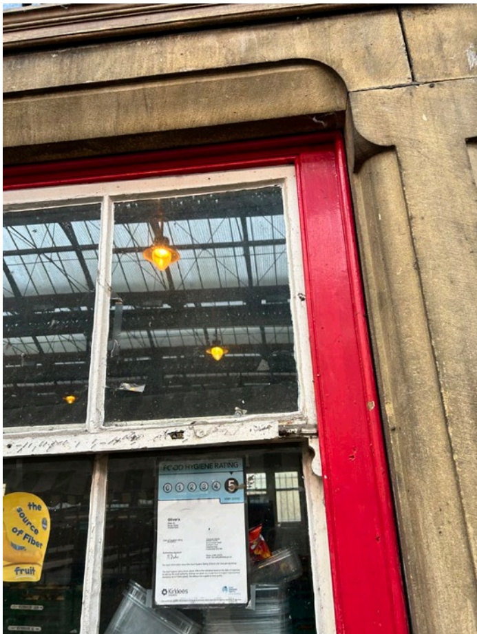
Photograph inside the existing market hall
