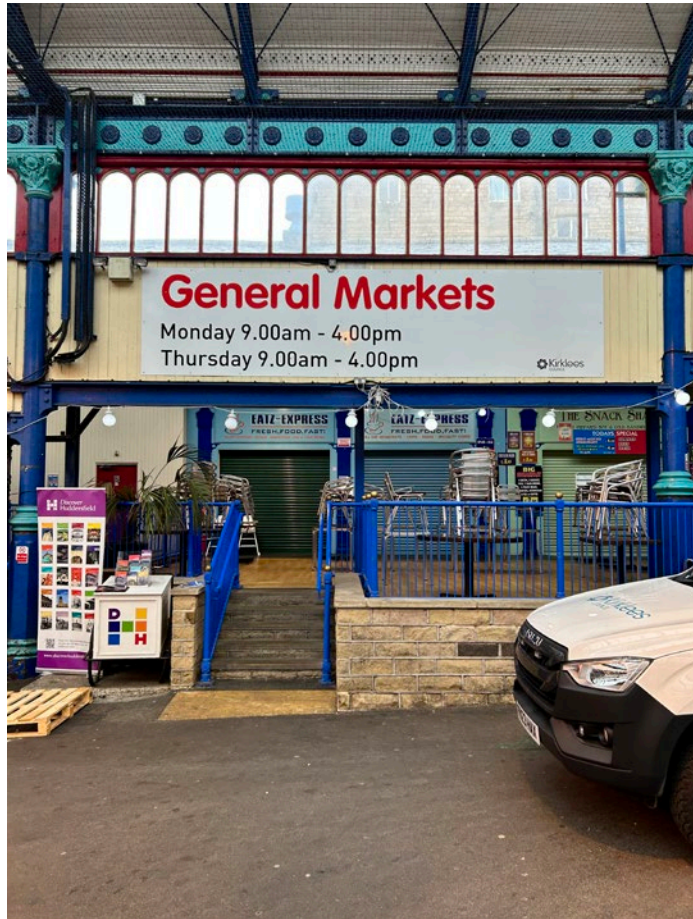
Photograph inside the existing market hall
