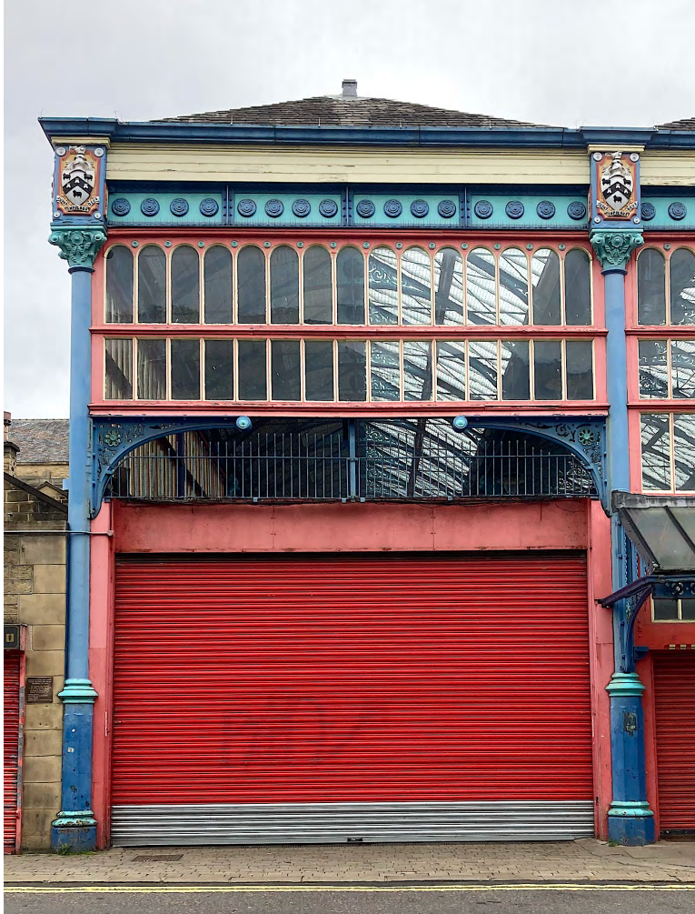
Figure 2: View of a single bay
