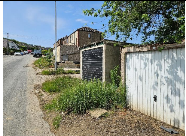
Photo 4: Building 1 and 2 on the developed land sealed surface.
