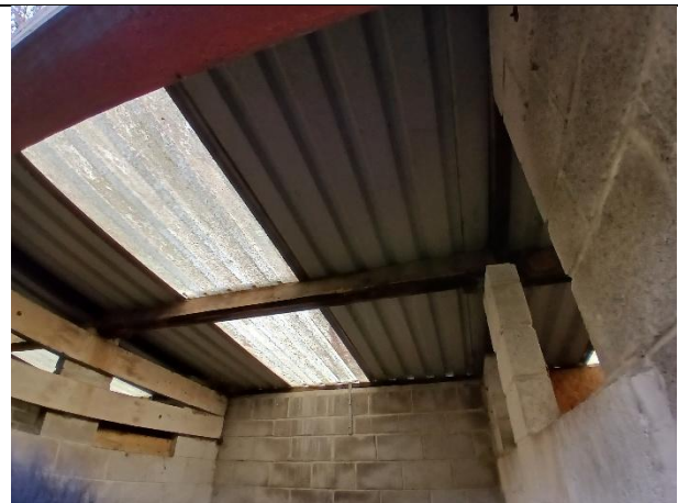
Photo 2: Inside of building 1.
