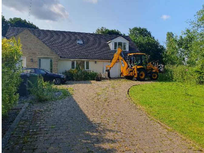
Looking south towards the detached house present on site.
