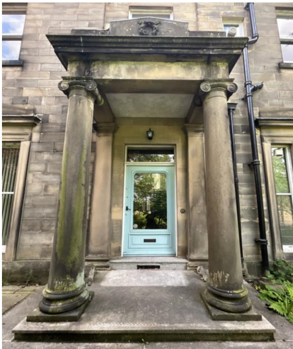
Figure 4: Grade II Listed Entrance Columns. View of the classical stone entrance portico, including the original columns which are Grade II listed. These features will remain entirely unaffected by the proposed change of use.
