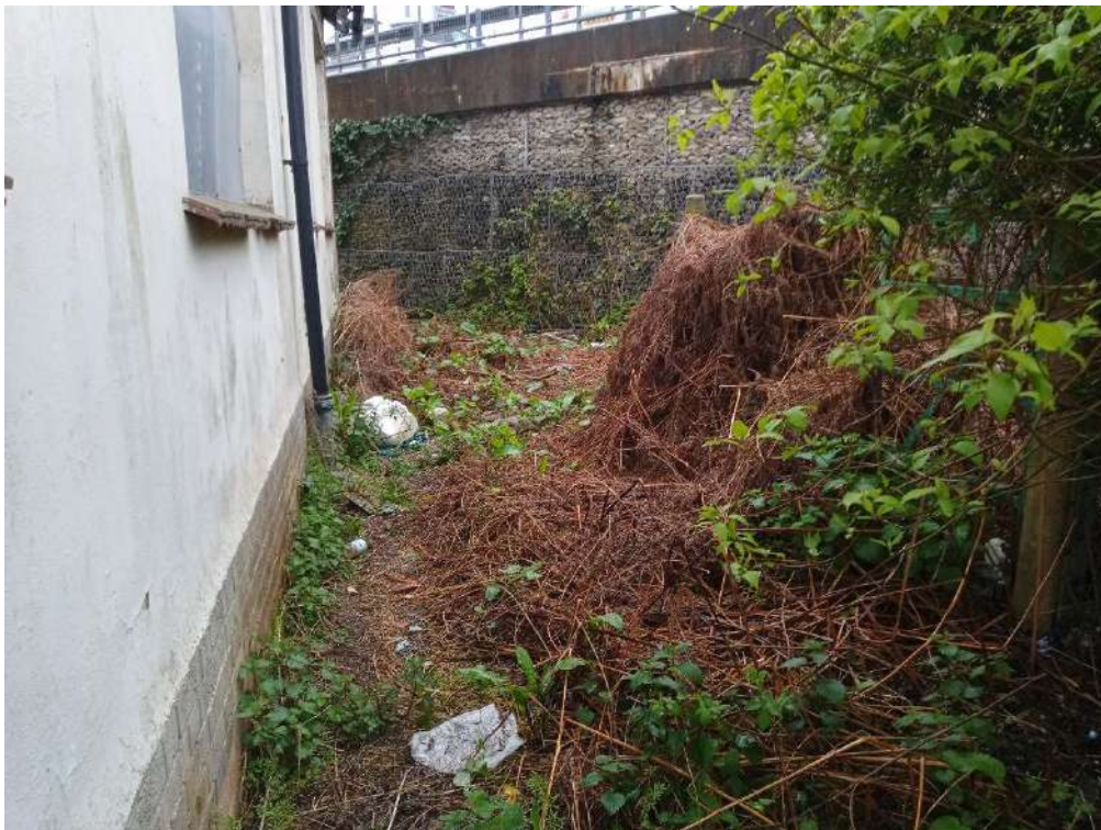
Side access and northern retaining wall with overgrown original substation and fence and possible tank bases
