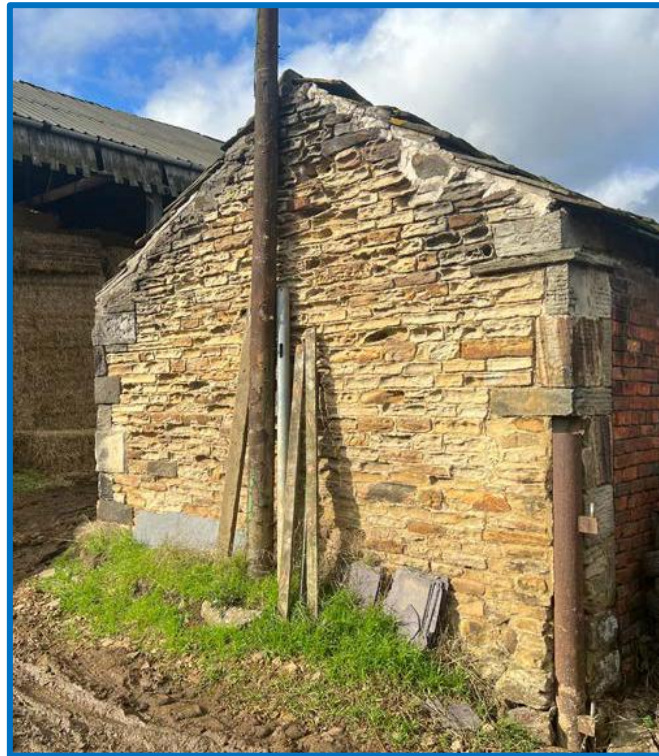
IMAGE 3 – CART SHED SOUTH FACING ELEVATION
