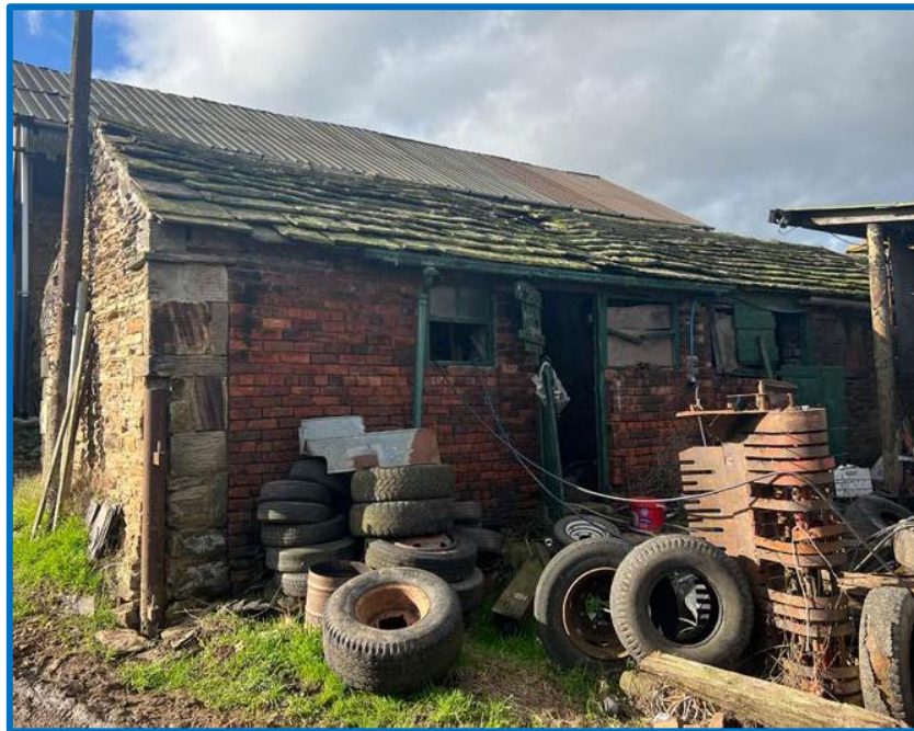
IMAGE 1 – CART SHED EAST FACING ELEVATION
